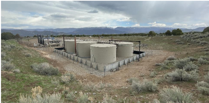
South West corner of location.
