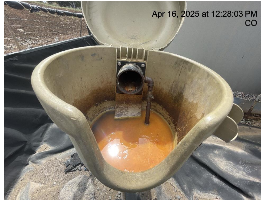
Photo # 1802 Open ended load line
