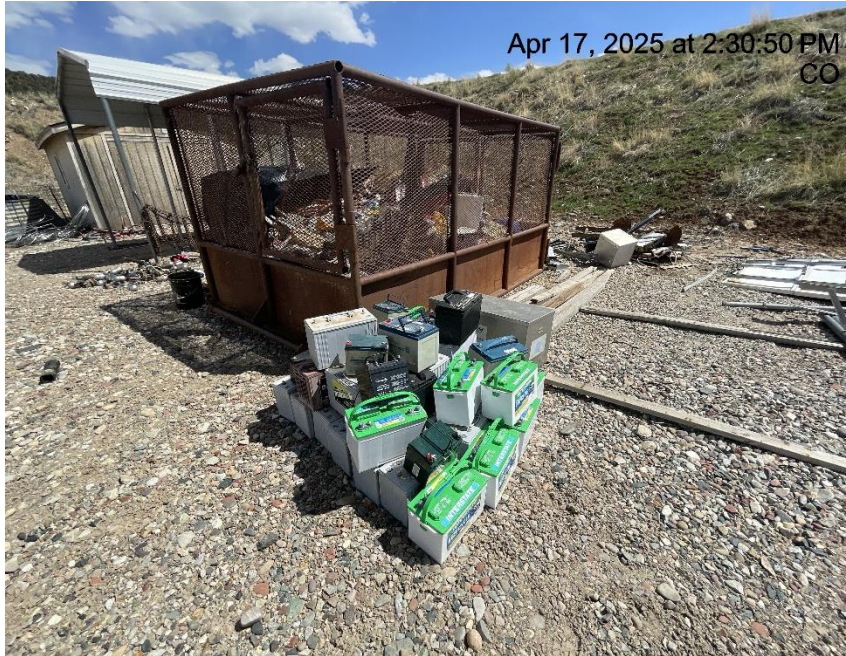
Photo # 2667 Batteries on location with no BMP's
