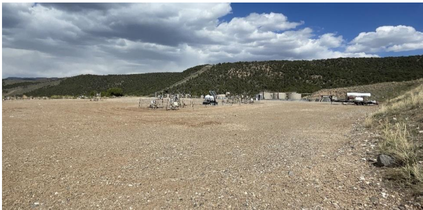
South West corner of location.
