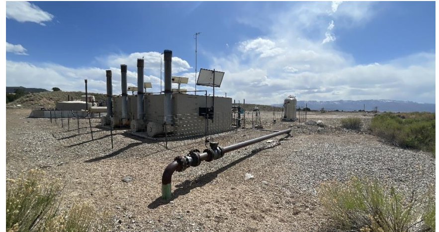
North East corner of location.
