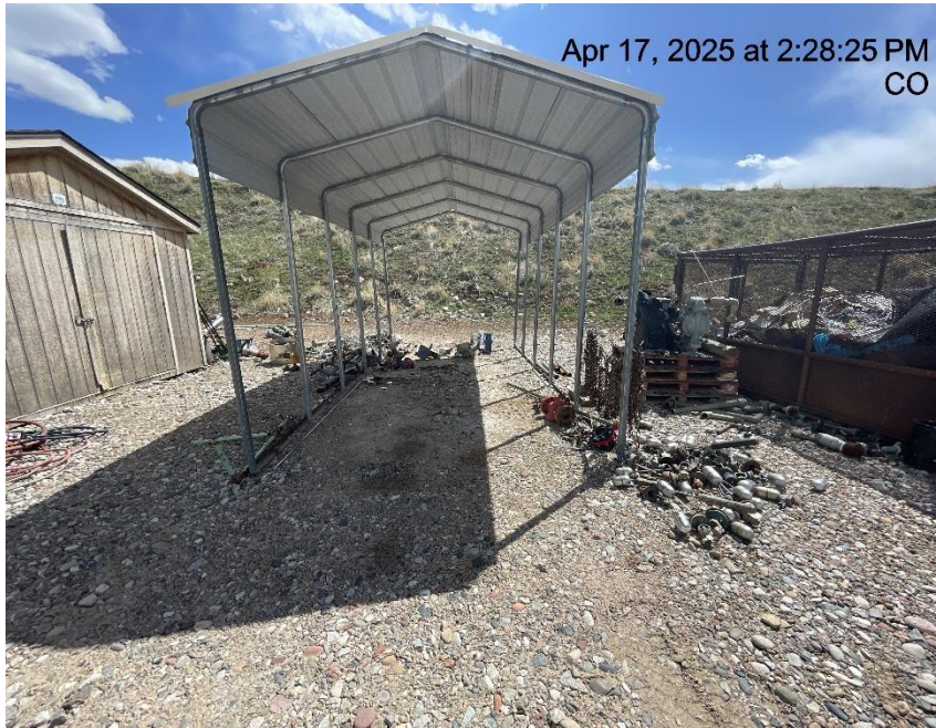
Photo # 2648 Carport on location/not in compliance with CECMC rules
