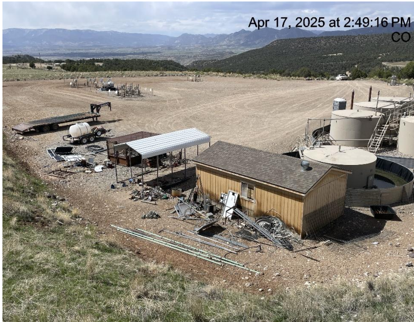
Photo # 2666 Unused equipment, stored supplies, trailers, carport, shed & misc
