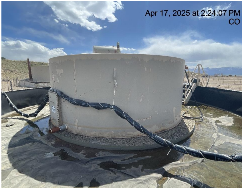
Photo # 2644 Arctictherm E-50 tank label lacks required information
