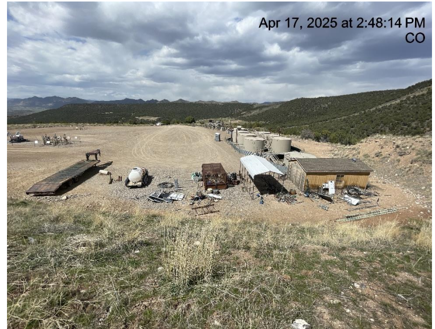
Photo # 2665 Unused equipment, stored supplies, trailers, carport, shed & misc
