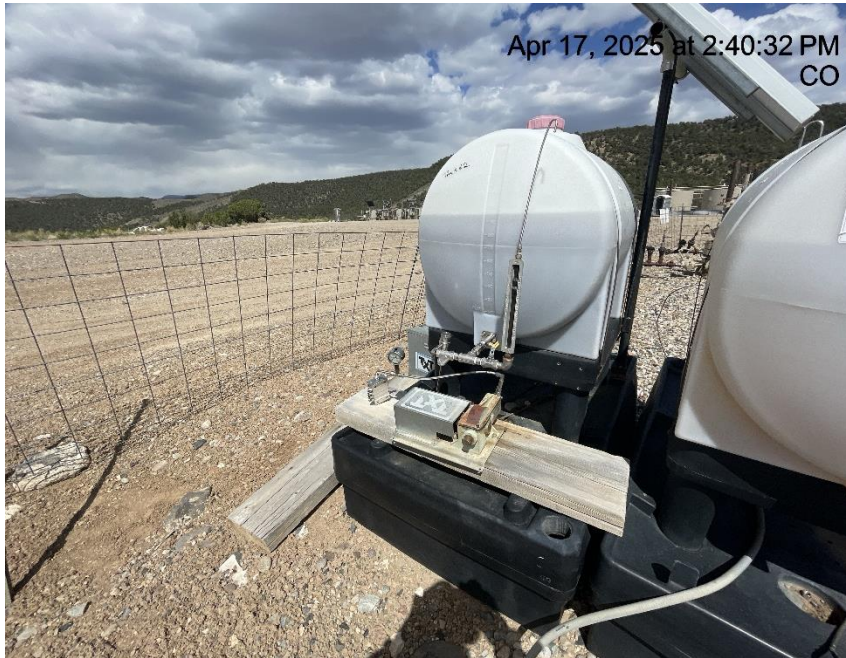
Photo # 2662 Unused chemical tank
