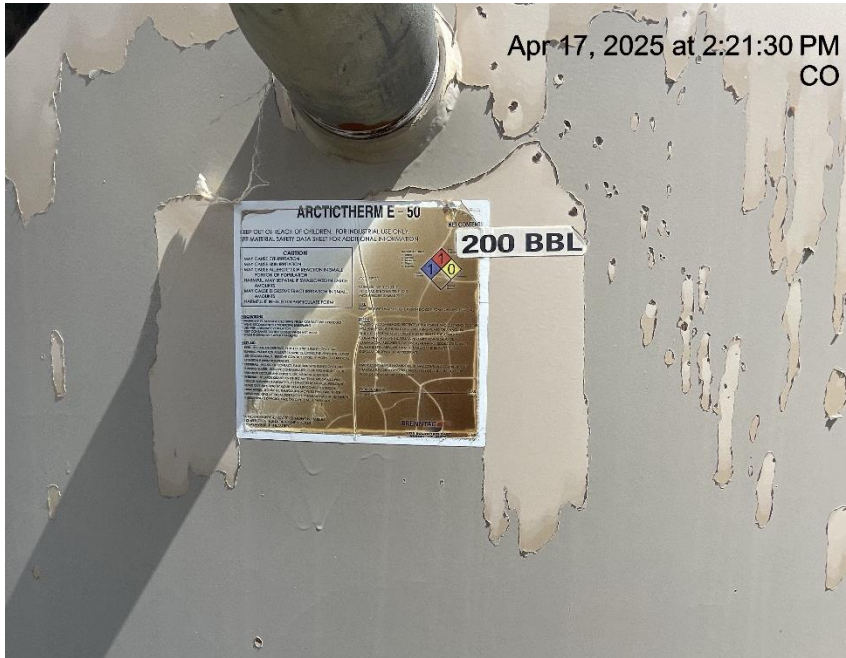
Photo # 2640 Arctitherm E-50 tank label lacks required information
