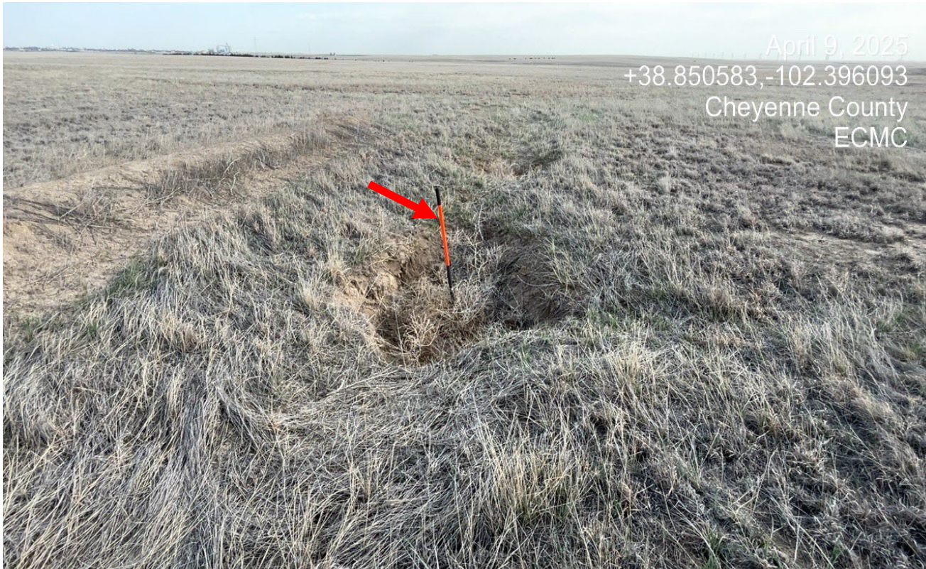
Photo 11. Facing south at the former pit area. There are two areas of subsidence at this former pit. Red arrow points to 4.5' shovel for scale.
