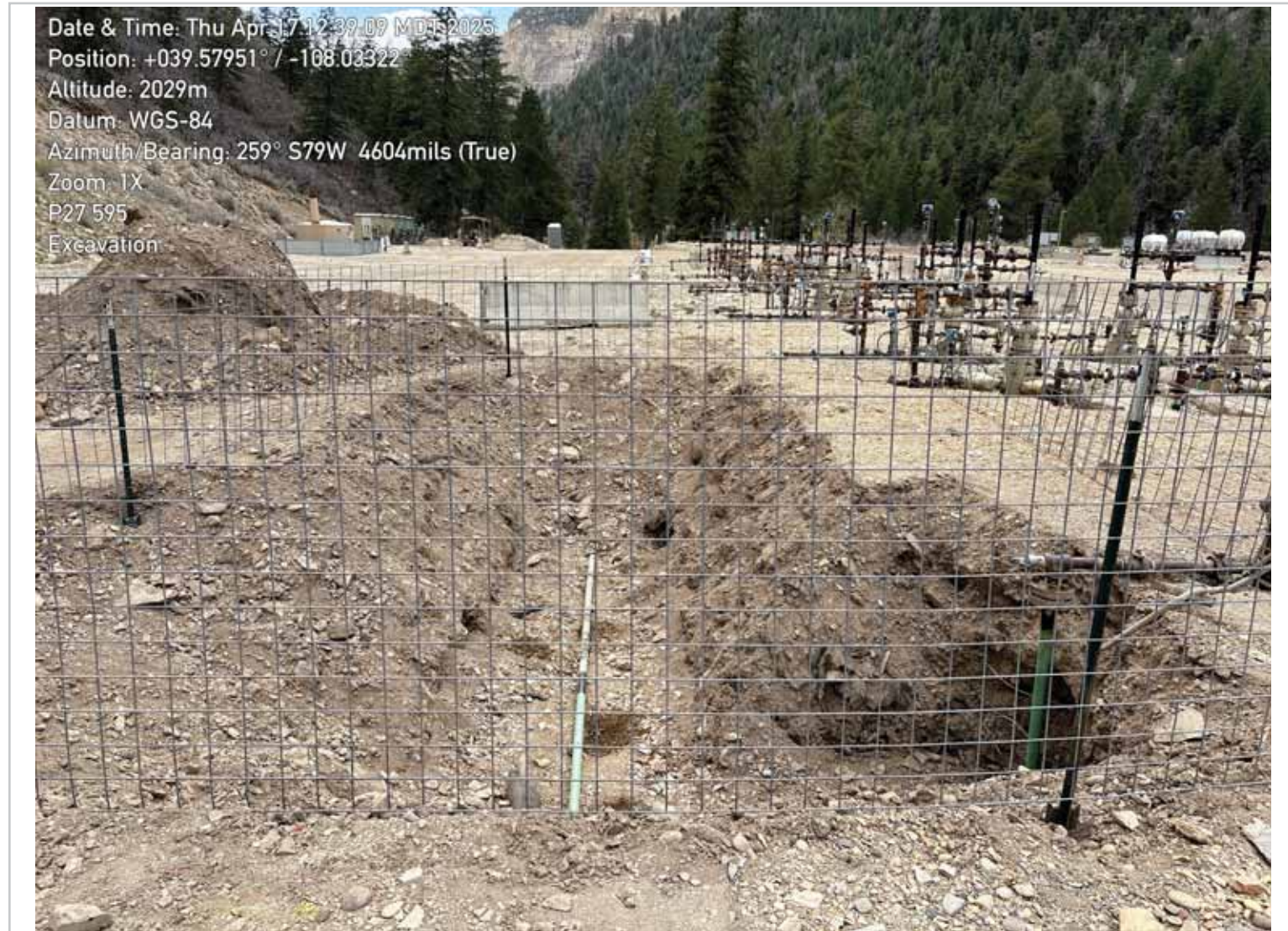
P27 595 16C-27 Excavation: View Southwest
