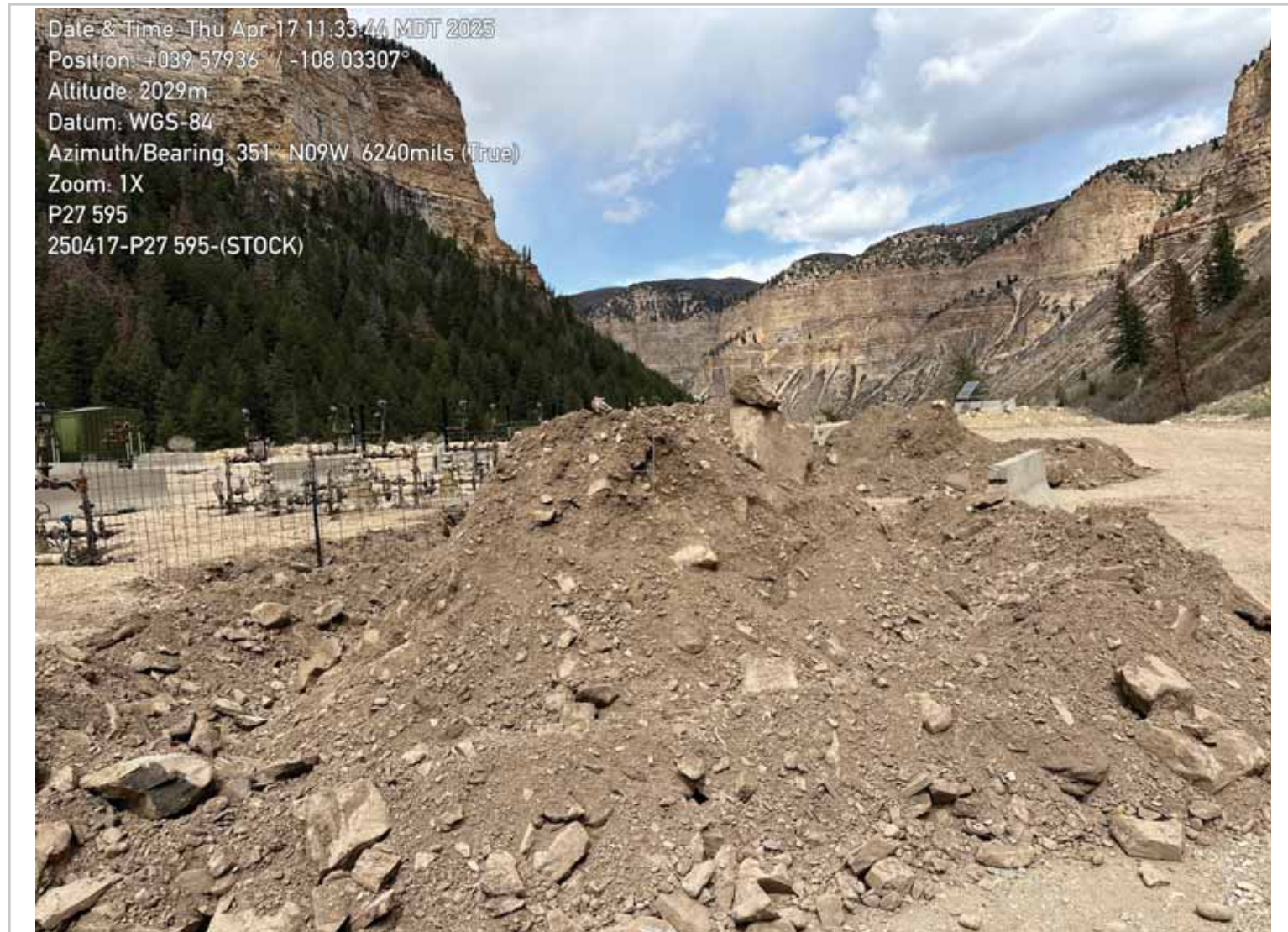
Soil Stockpiles: View Northwest
