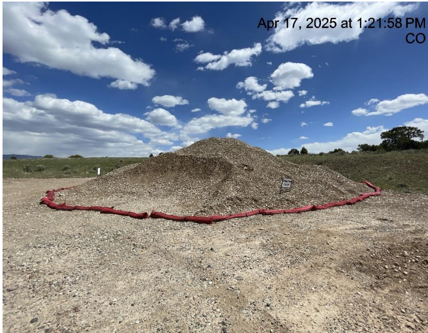
Photo # 2496 Stockpiled soils & gravel with BMP's
