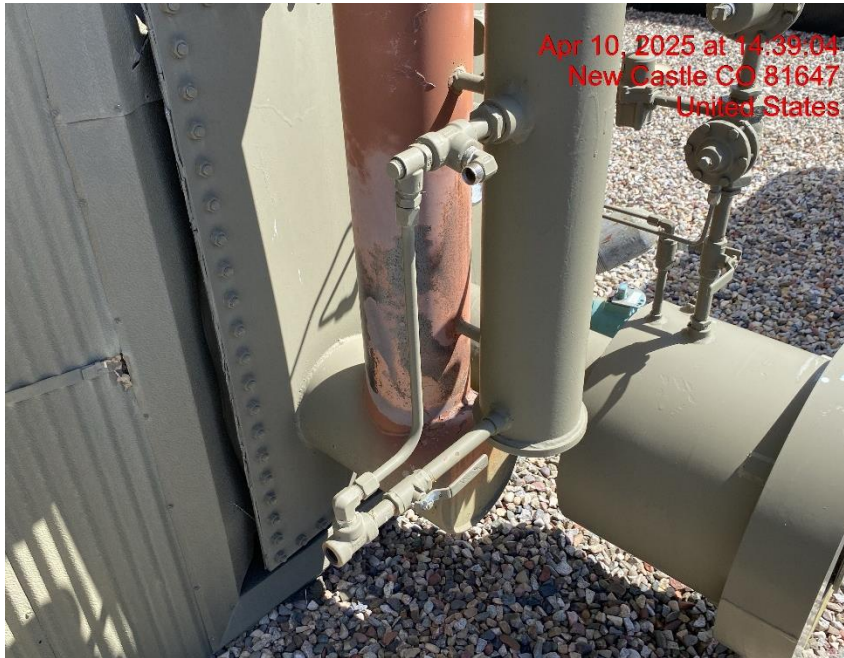
PRV Terminates in Unsafe Manner – Photo #08079
