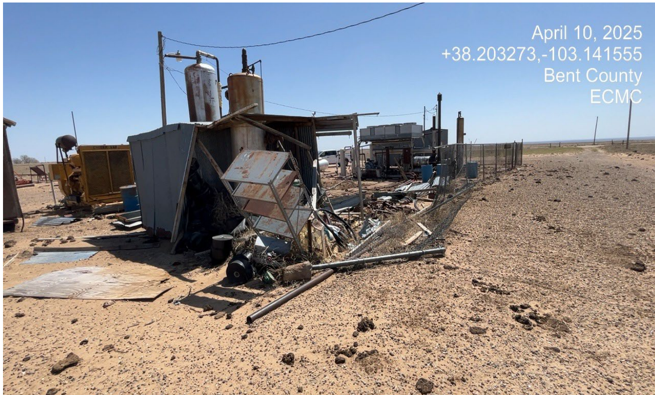
Photo 9. Facing southeast at the west side of the location. This shed and fence are in disrepair with supplies have fallen out of the dilapidated shed.
