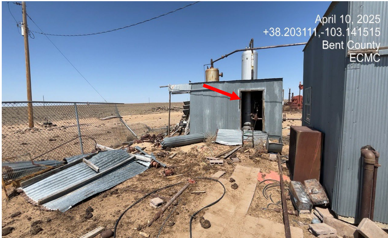
Photo 8. Facing northwest at the sheds and equipment which are in disrepair. There was an audible gas leak coming from this shed and separator shown at red arrow.
