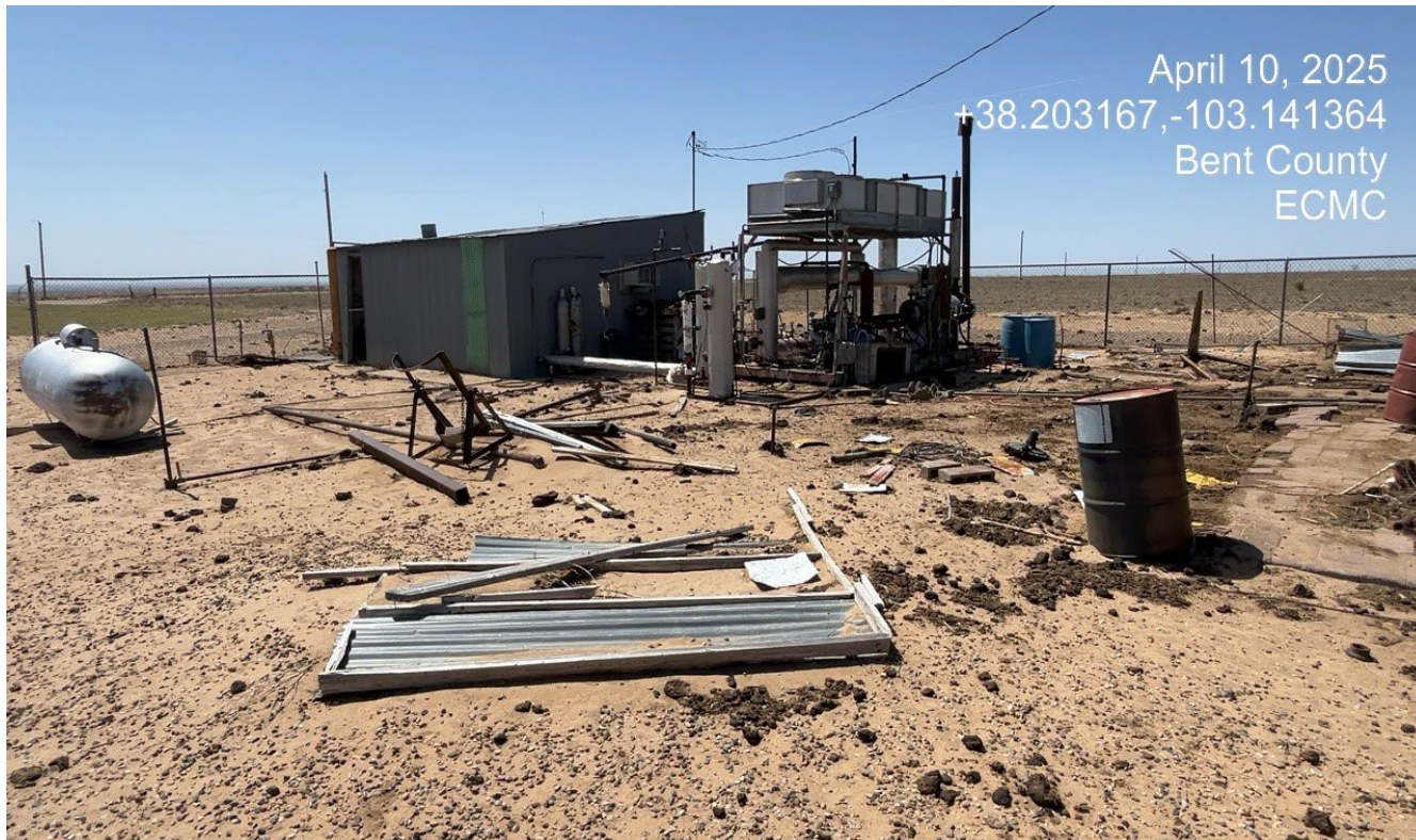
Photo 4. Facing southwest at the sheds and various equipment which are in disrepair. There is chemical barrels with no containment and various debris laying on the ground.
