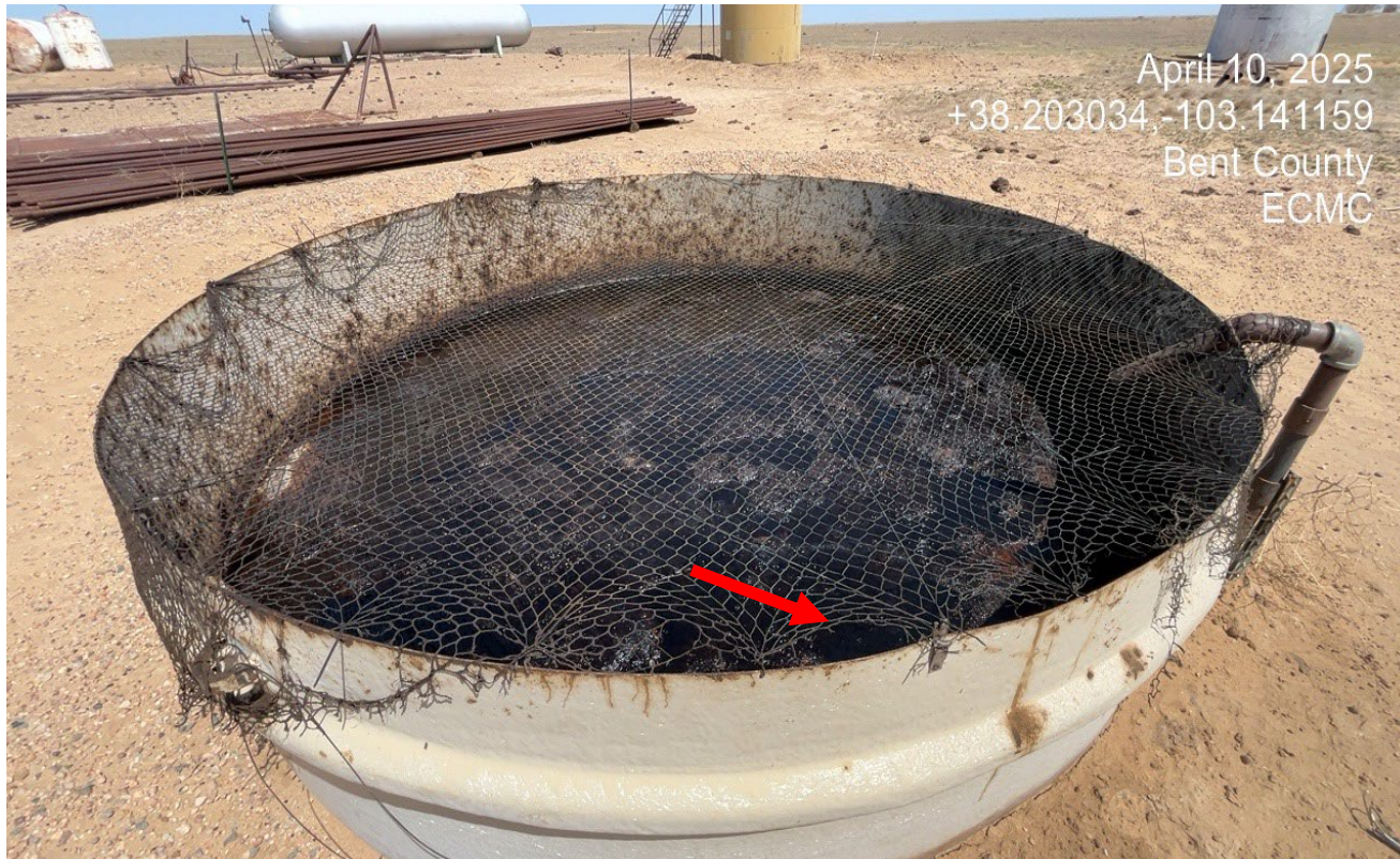
Photo 15. Facing toward the open top tank which has oil condensate inside the tank. Netting has now been installed over the tank. There are still opening on the sides that are large enough for birds to get into the tank.
