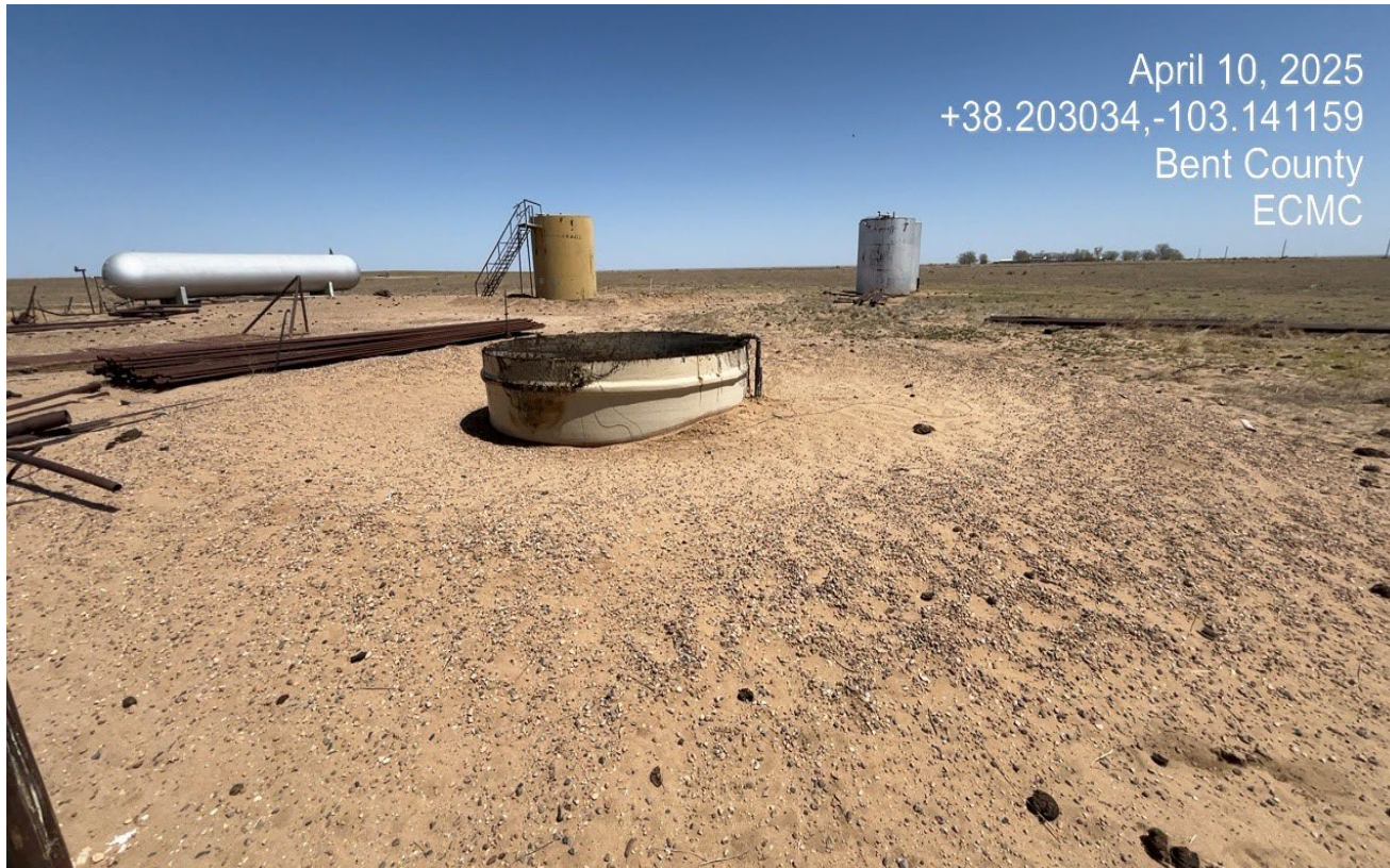
Photo 14. Facing east at the south side of the location. This open top tank remains with oily fluids.
