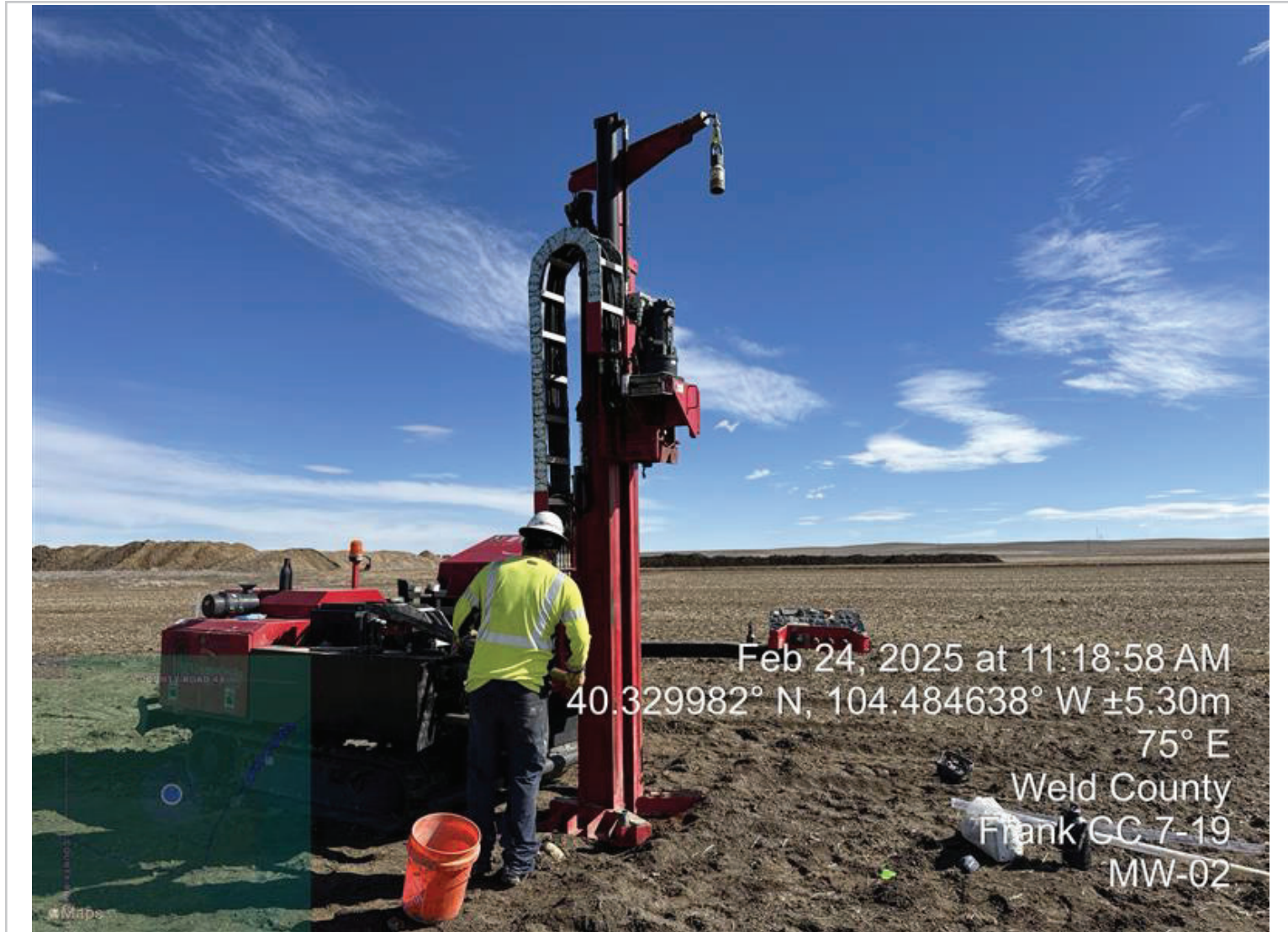
Soil Boring Location MW-02: View East
