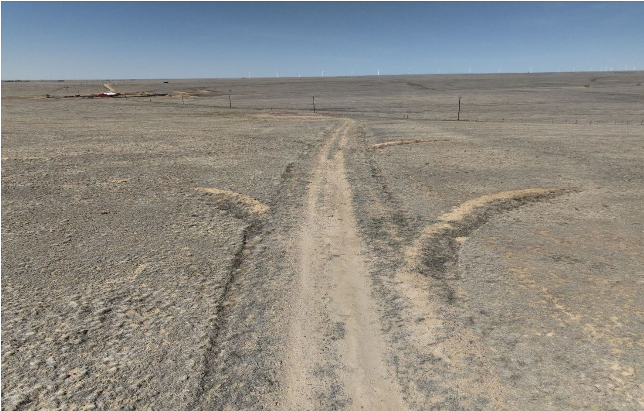
Photo 2. Drone aerial photo facing west toward the access road. The access road has not been recontoured and reclaimed which include the diversion ditches.
