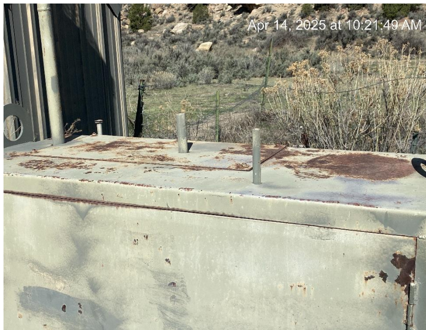
Unprotected relief vent risers
