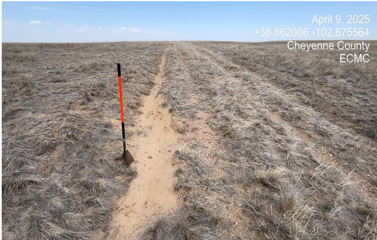
Photo 1. Facing northeast along the two track access road. There is an erosion channel along the road closer to the location that needs to be repaired.
