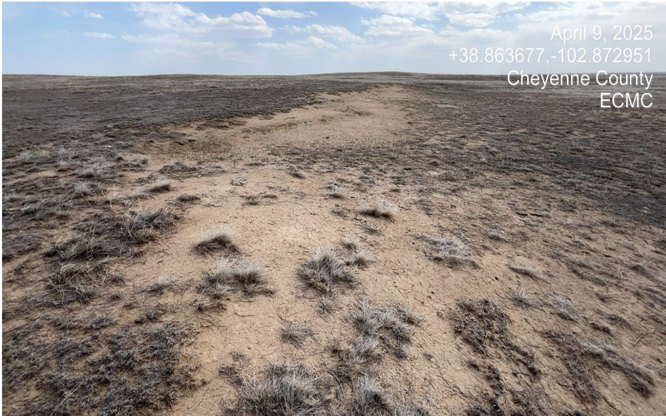
Photo 6. Facing south along the cut slope. The cut slope is approximately 2-3 ft. and needs to be resloped with topsoil and revegetated.
