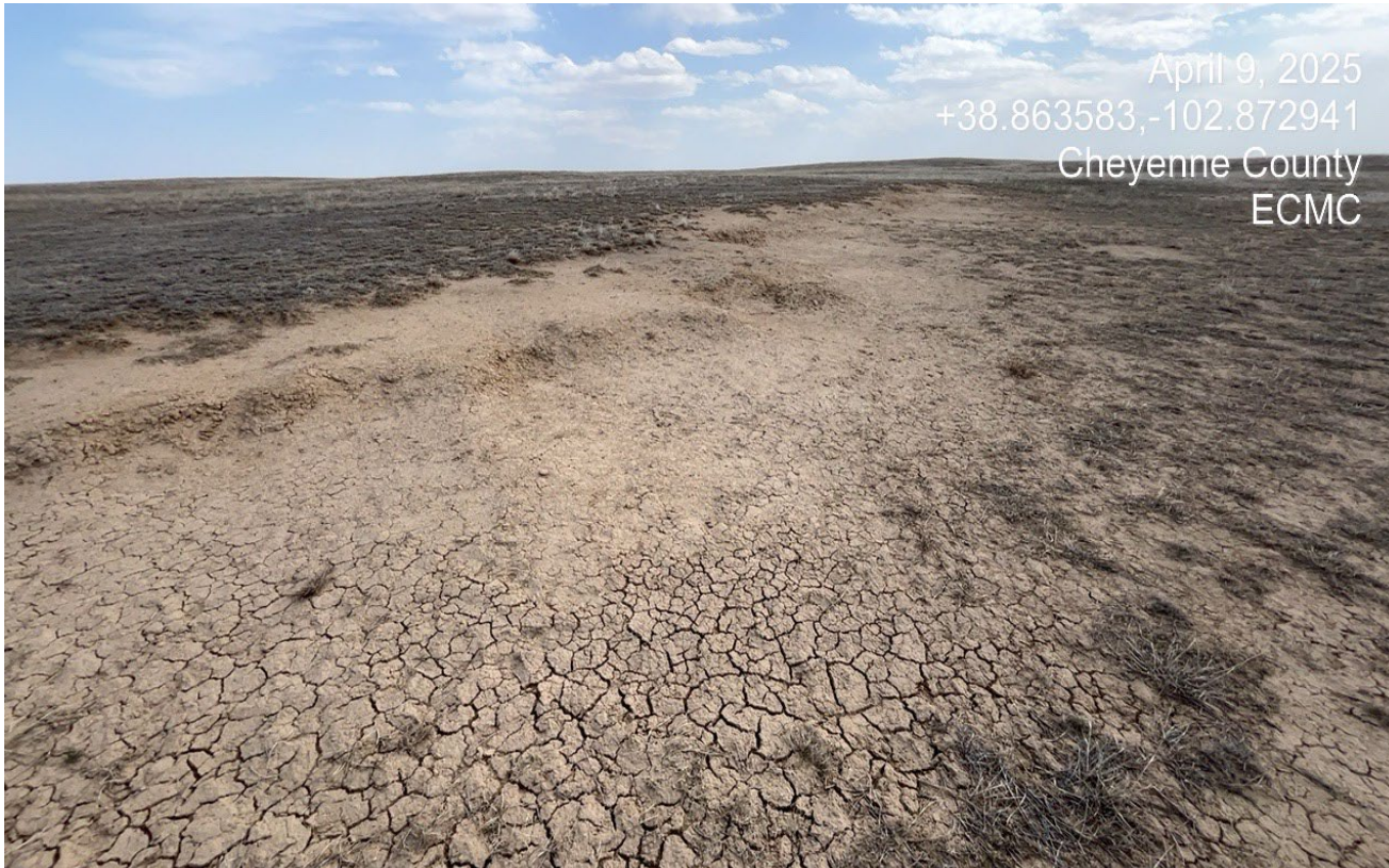
Photo 7. Facing south along the cut slope. The cut slope is approximately 2-3 ft. and needs to be resloped with topsoil and revegetated.
