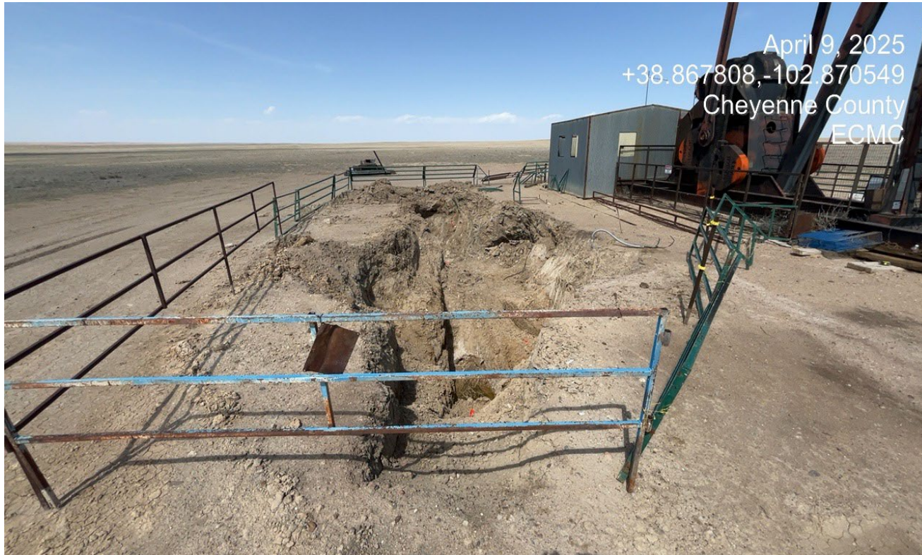
Photo 5. There is open excavation of active remediation from previous spill observed.
