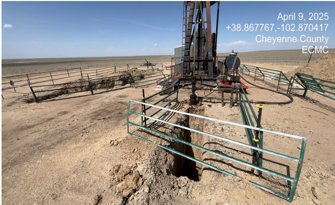
Photo 4. There is open excavation of active remediation from previous spill observed.
