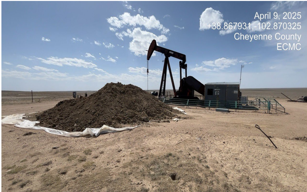
Photo 6. The impacted soils are not being stored with containment and have spread off of the plastic liner.
