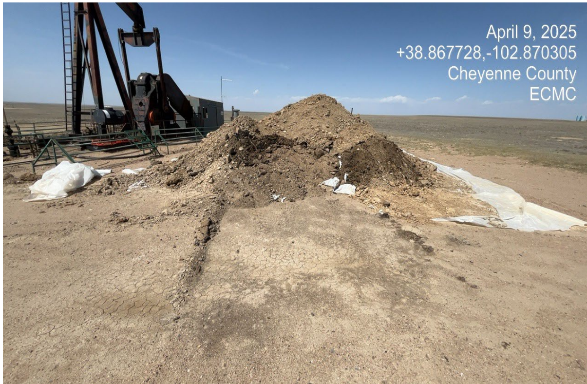
Photo 3. The impacted soils are not being stored with containment and have spread off of the plastic liner.
