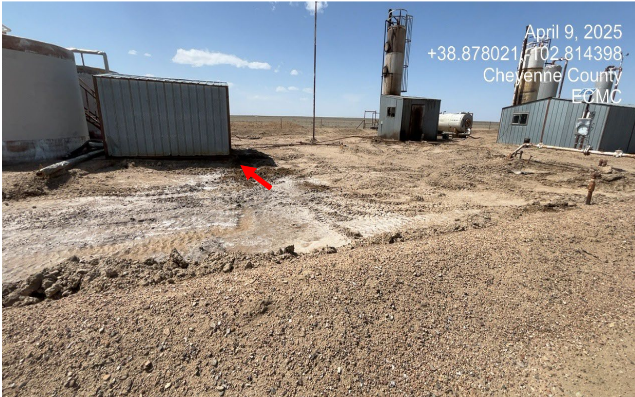
Photo 5. It appears there was also a condensate leak that flowed from the shed at red arrow.
