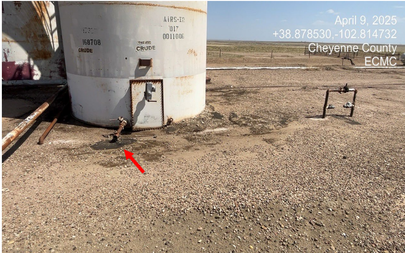
Photo 2. Facing northeast toward the tank battery. The oil stained waste remains around the tanks. Some of the tanks were removed since the previous inspection.
