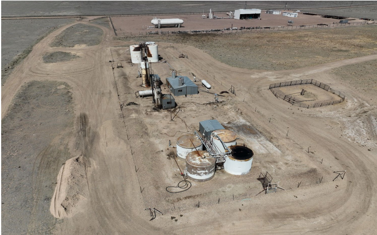
Photo 7. Drone aerial photo facing northeast toward the tank battery facility.
