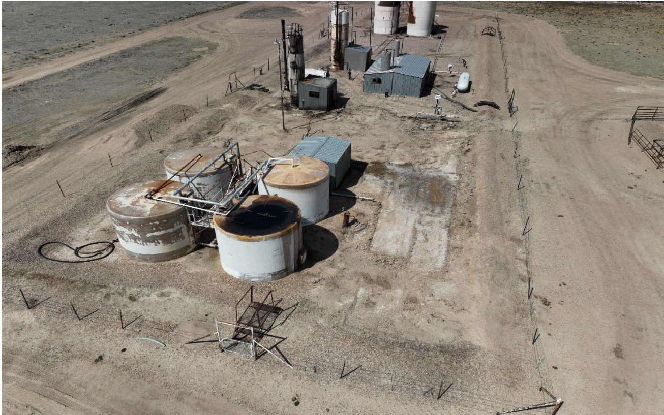
Photo 8. Drone aerial photo facing northwest toward the tank battery facility. The previous spill that occurred flowed to this southeast corner and overtopped the berm.
