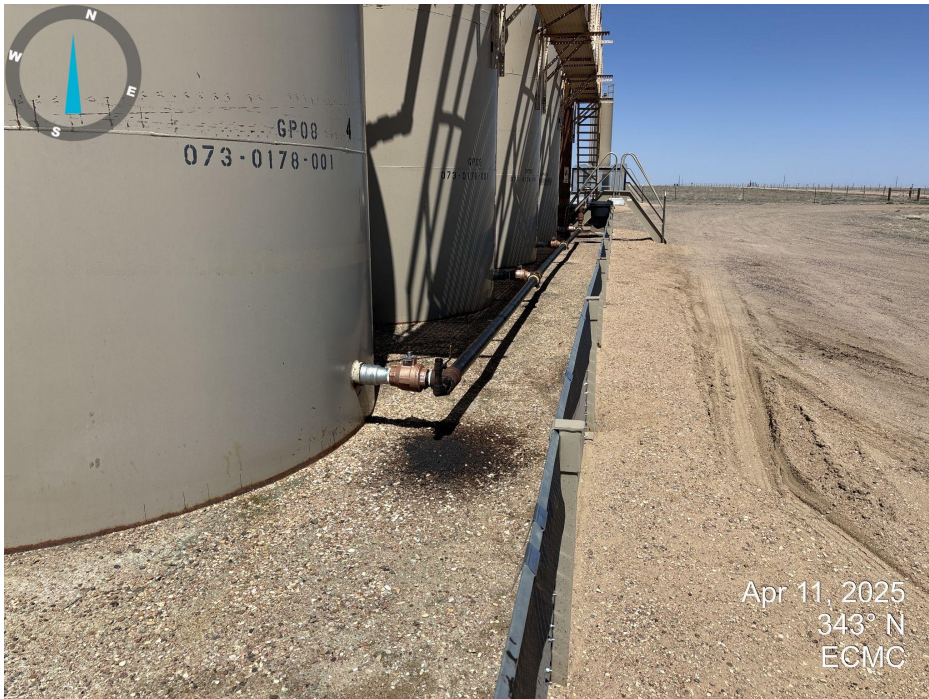
Photo 3. Stained soil beneath valve on the east side of southern tank.
