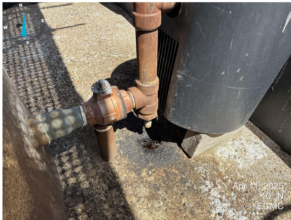
Photo 8. Picture taken on the east side of the northern fiberglass tank. Stained soil beneath valve.
