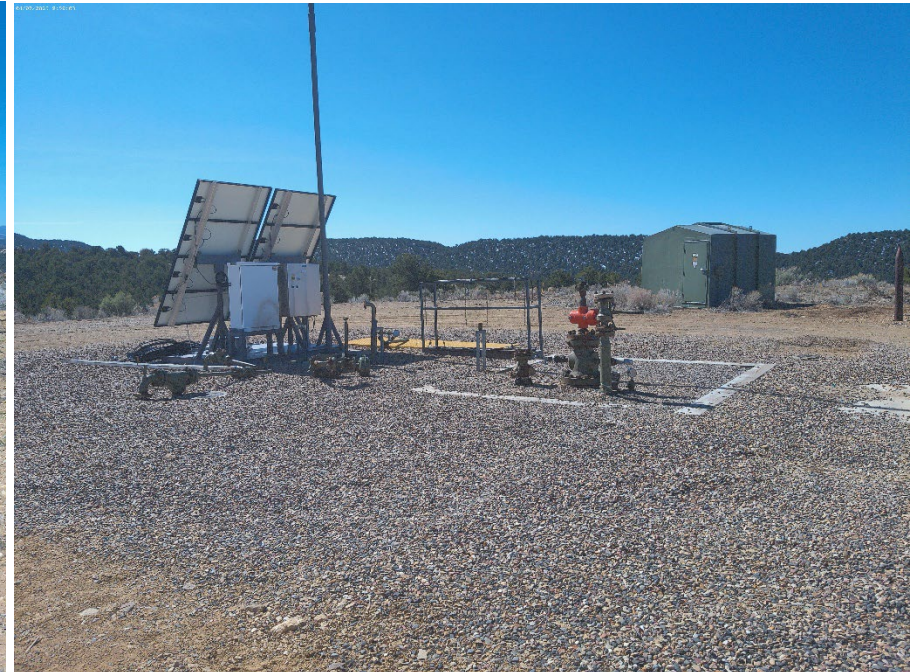
Injection Wellhead
