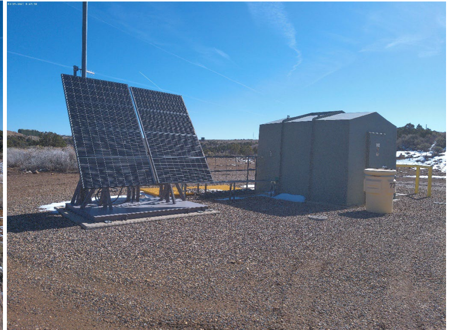
Injection Wellhead inside housing
