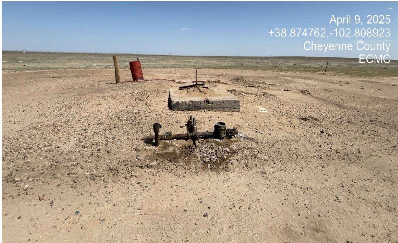
Photo 4. Facing toward the wellhead. There are stained soil at the wellhead. This area will need to be sampled and remediated for decommissioning of the well.
