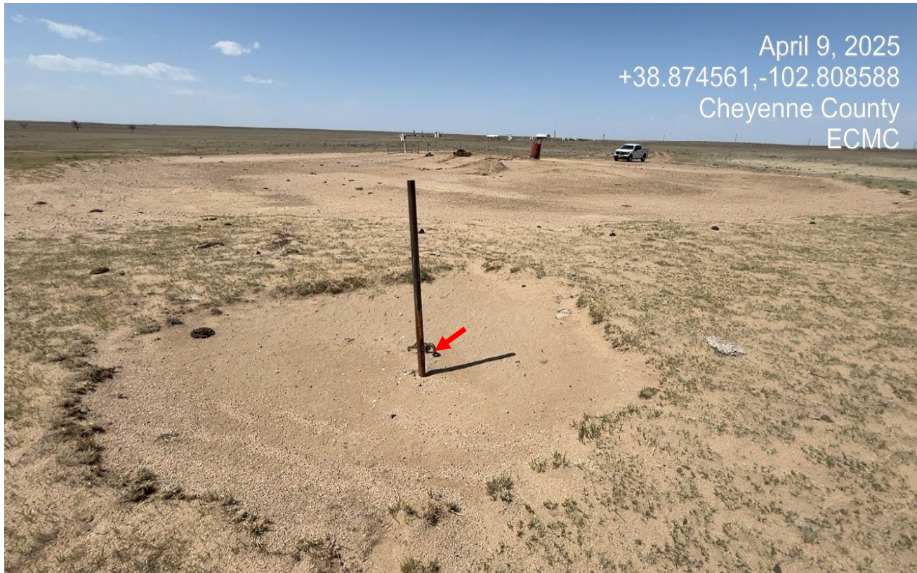
Photo 6 . There are 4 guyline anchors that remain at the location that must be removed within 3 months of abandonment
