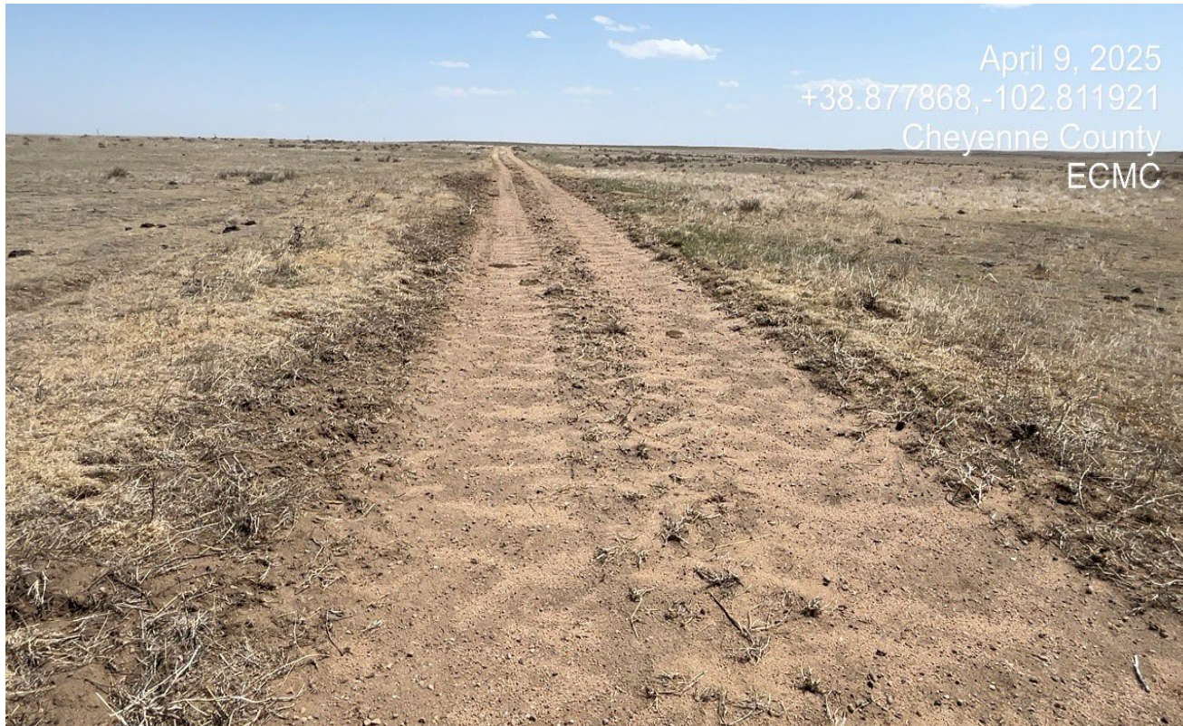
Photo 1. Facing southeast toward the access road. The access road is eroded and will need to be regraded to match the surrounding contours which may require imported topsoil.
