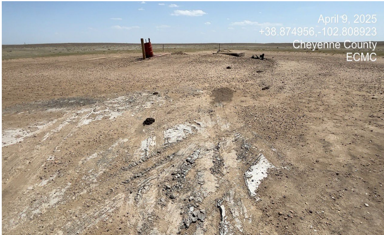
Photo 3. There is stained soils and cement spilled on location that will need to be cleaned up. Previous CA was not completed.
