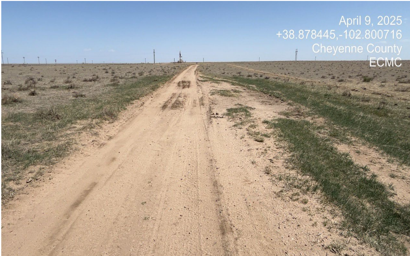
Photo 14. Facing east along the access road. Vehicles are causing unnecessary disturbance driving outside of the access road due to stormwater pooling on the road. The access road must be maintained and shall not drive outside of the access road boundary.
