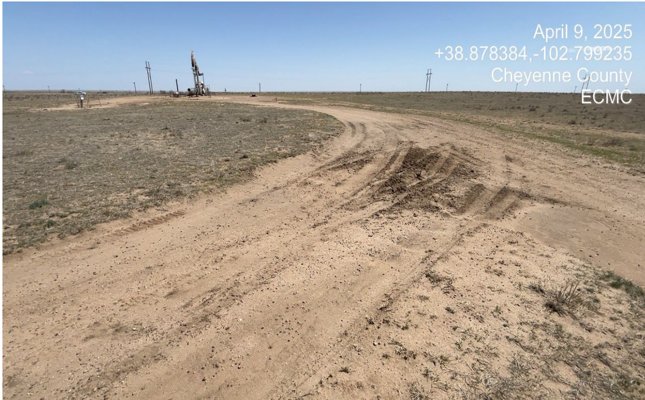
Photo 2. Facing southeast along the access road. The access road has not been repaired and stabilized. This is a low spot of the road where stormwater accumulates.
