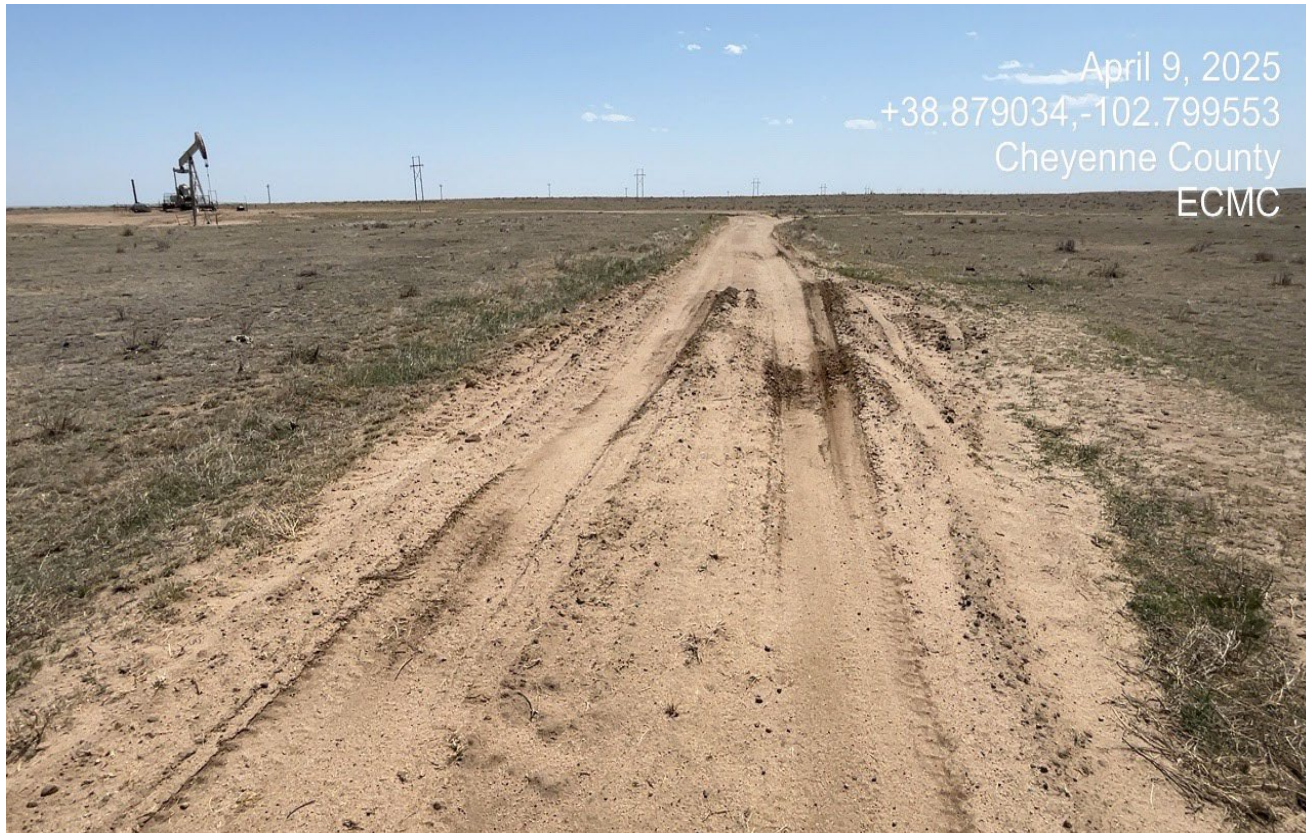
Photo 1. Facing south along the access road. The access road has not been repaired and stabilized. This is a low spot of the road where stormwater accumulates. It does not appear vehicles have been driving outside of this area recently.
