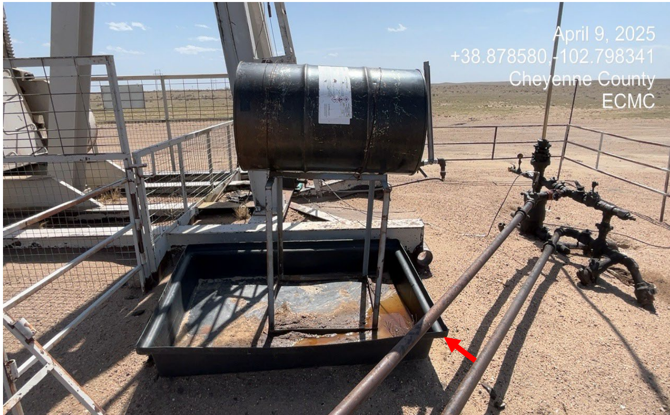
Photo 7. This chemical drum has been placed in secondary containment. The containment has oily fluids and needs to be covered/netted to prevent wildlife entry.
