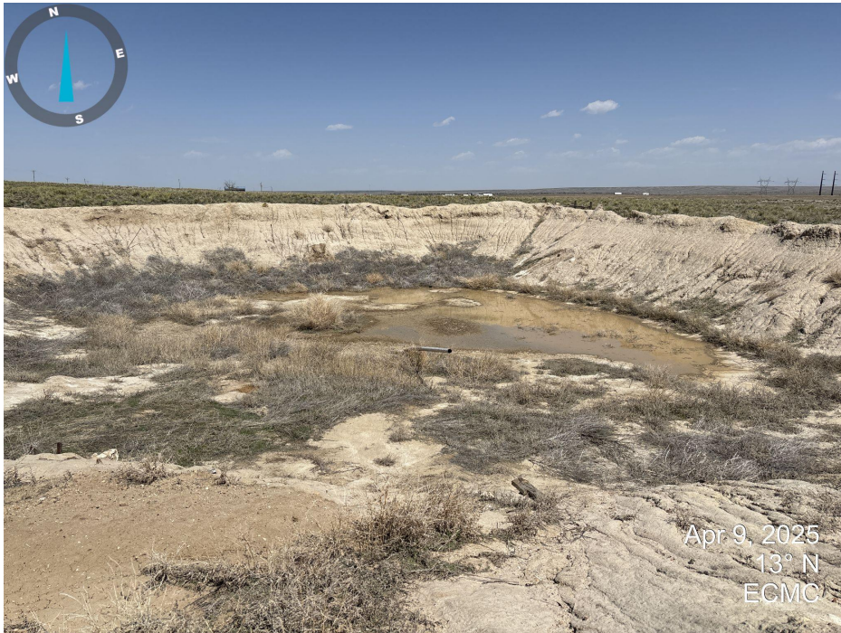
Photo 13. Looking north across evaporation pond. Channel erosion is present around the entire interior of the pond. Standing water is present in pond at the time of inspection.
