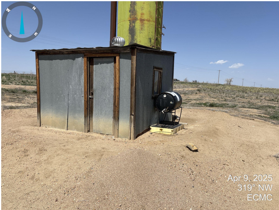
Photo 9. Looking northwest at the separator shed. Barrel secondary containment does not have a wildlife exclusion device installed.
