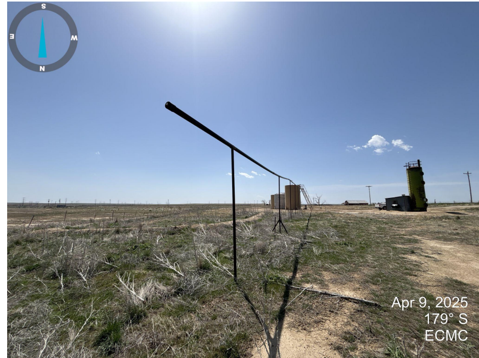
Photo 12. Pipe from produced water tank to evaporation pond is capped off.
