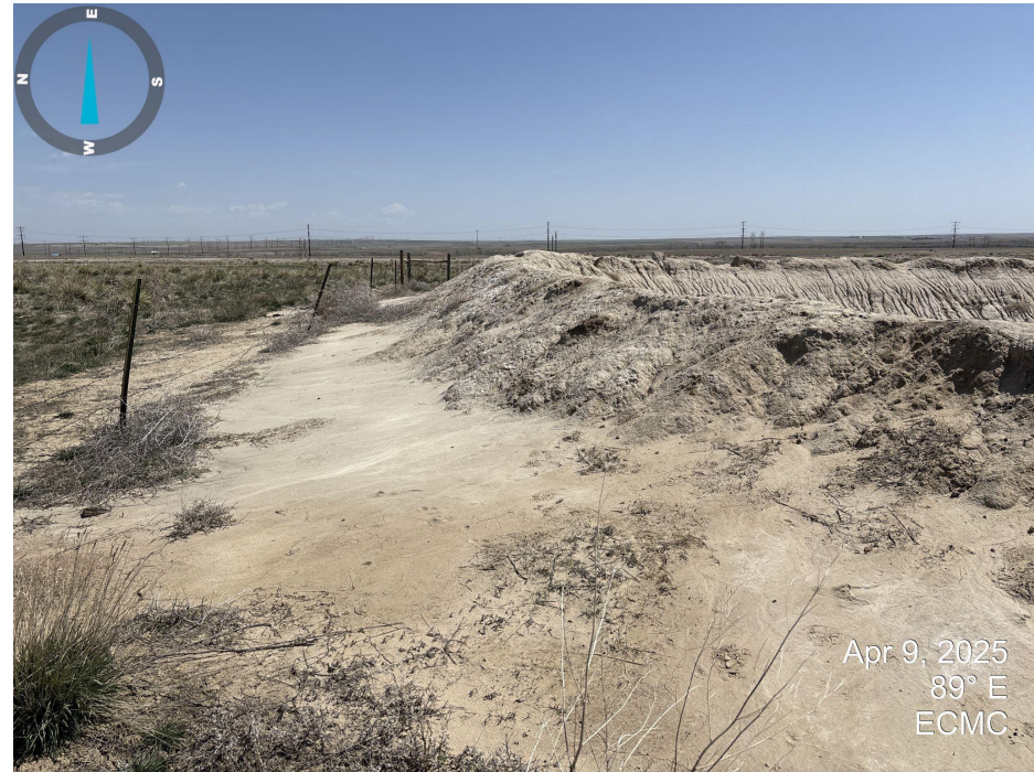
Photo 14. Looking east long north side of pond. Heavy erosion is present on the outside of the berm and sediment is being transported off location by stormwater.
