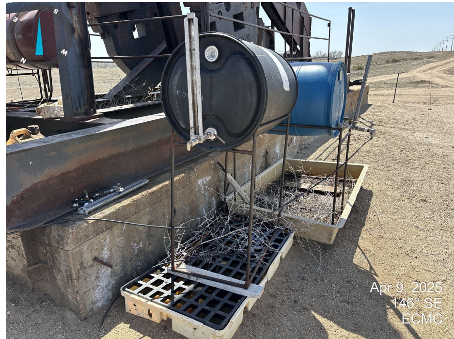
Photo 8. Barrels on the west side of location. Secondary containment does not have wildlife exclusion devices.
