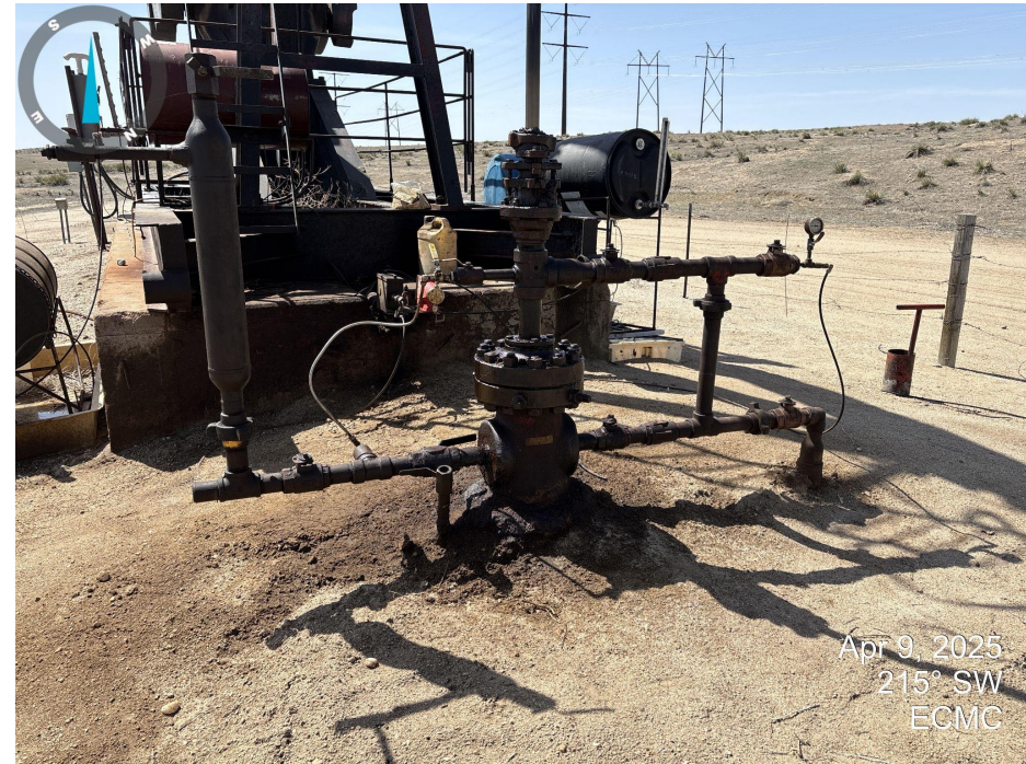
Photo 6. Wellhead appears to be leaking and stained soil is present around the base.
