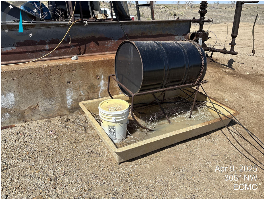
Photo 7. On the east side of location. An unmarked barrel. Secondary containment does not have wildlife exclusion device.
