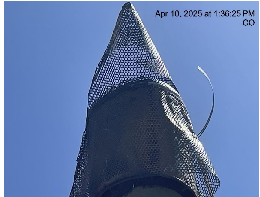
Photo # 396 Bird protection damaged & needs maintenance /wildlife hazard
