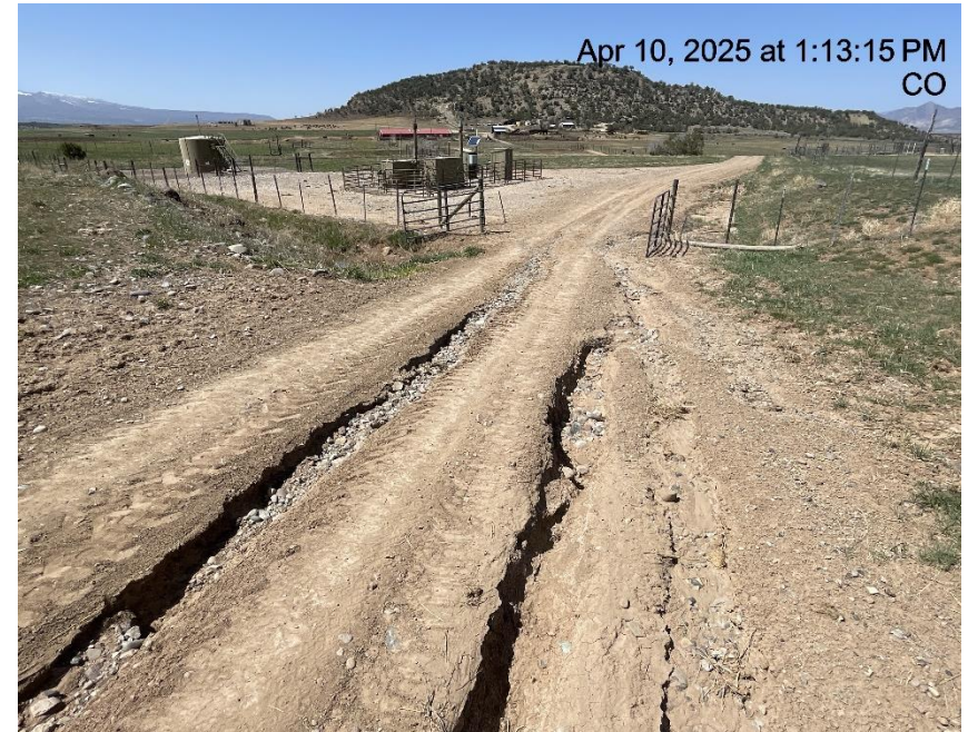
Photo # 99 Failure to minimize erosion & transport of sediment on lease road/road degradation
