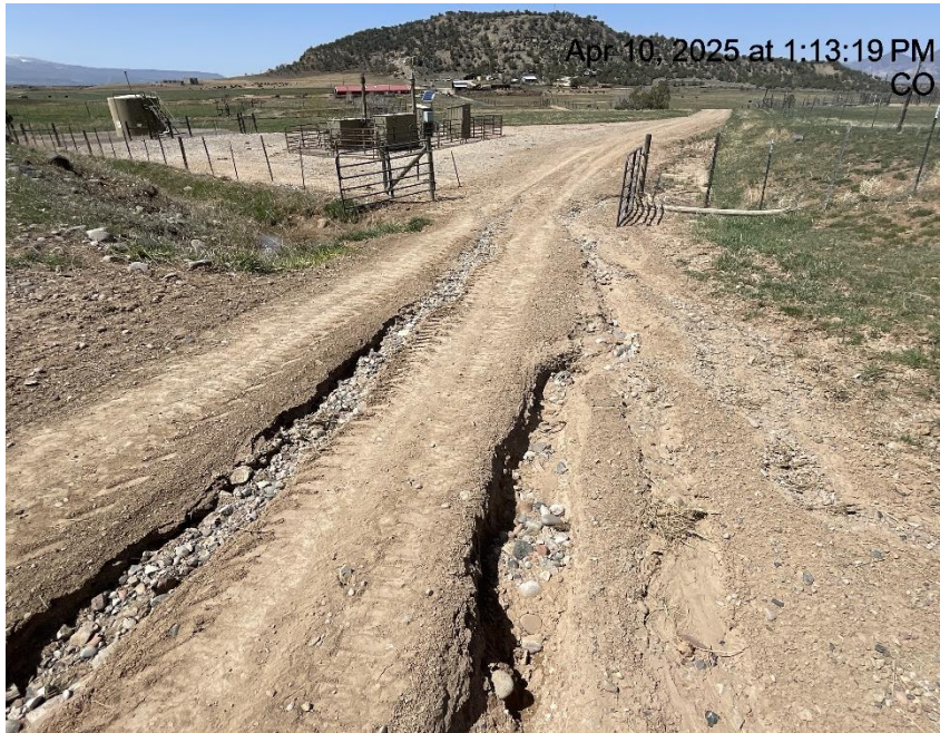
Photo # 100 Failure to minimize erosion & transport of sediment on lease road/road degradation
