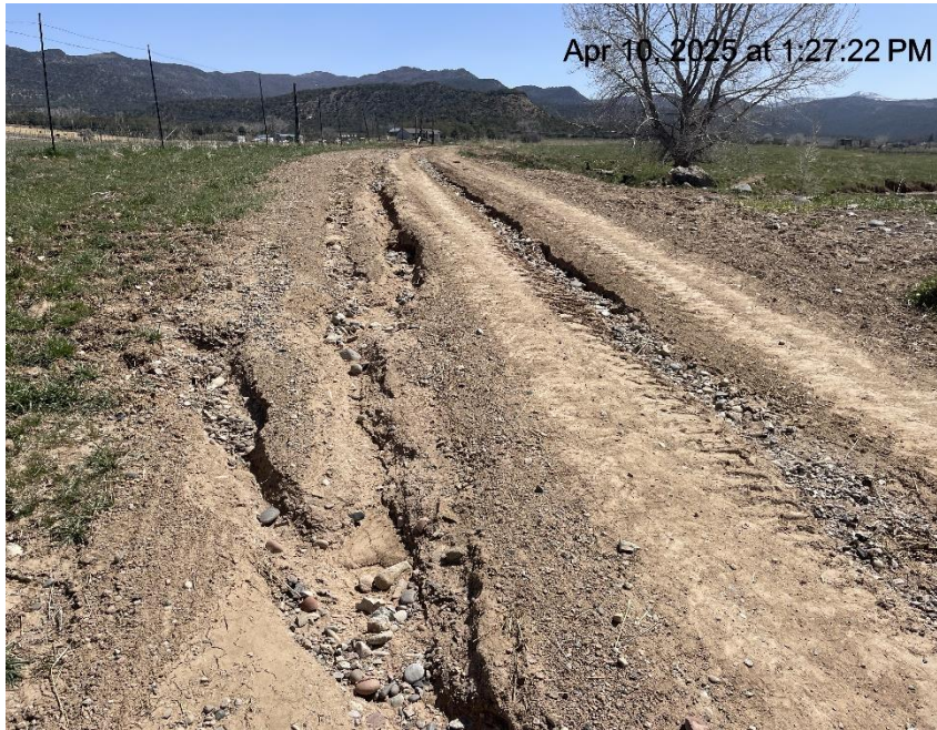
Photo # 96 Failure to minimize erosion & transport of sediment on lease road/road degradation
