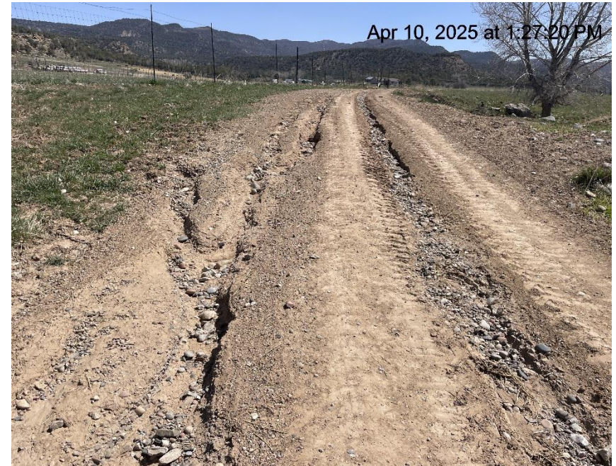
Photo # 95 Failure to minimize erosion & transport of sediment on lease road/road degradation
