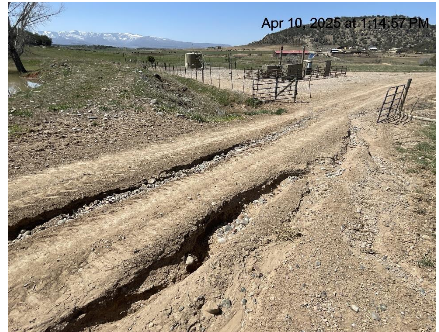
Photo # 101 Failure to minimize erosion & transport of sediment on lease road/road degradation
