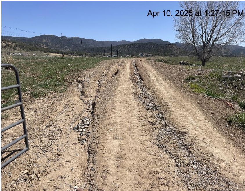
Photo # 94 Failure to minimize erosion & transport of sediment on lease road/road degradation
