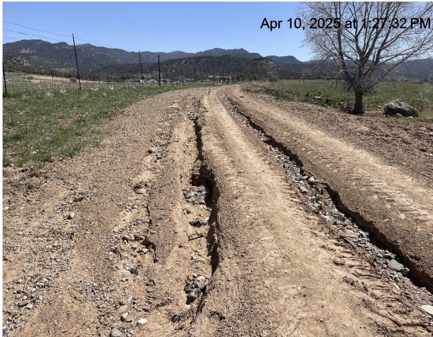
Photo # 98 Failure to minimize erosion & transport of sediment on lease road/road degradation
