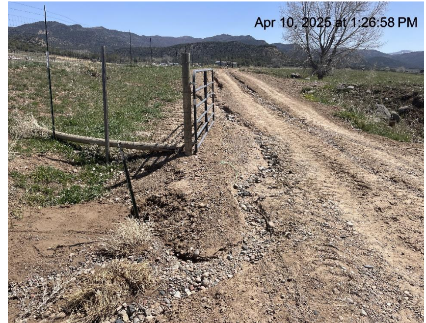
Photo # 93 Failure to minimize erosion & transport of sediment on lease road/road degradation
