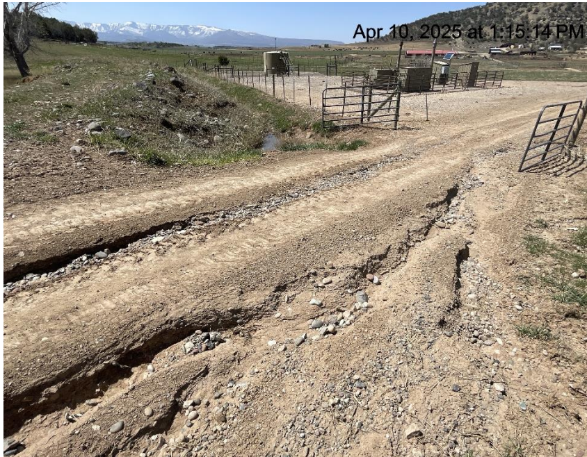
Photo # 102 Failure to minimize erosion & transport of sediment on lease road/road degradation
