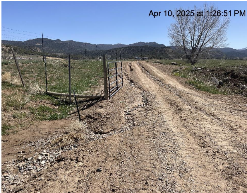
Photo # 92 Failure to minimize erosion & transport of sediment on lease road/road degradation
