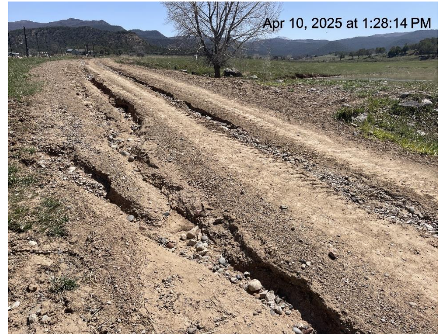
Photo # 97 Failure to minimize erosion & transport of sediment on lease road/road degradation
