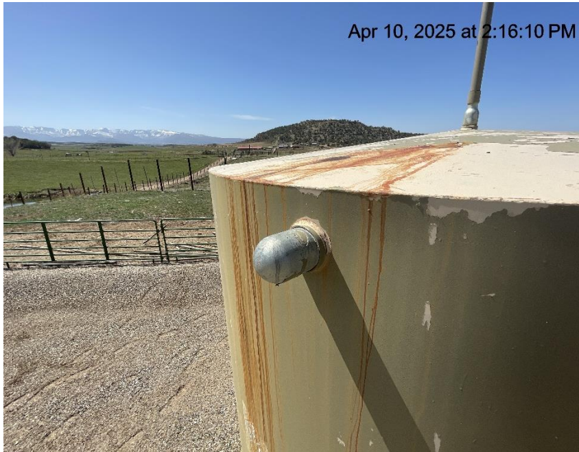
Photo # 480 Staining on top of tank & down the side of tank that indicates the tank may lack integrity.
