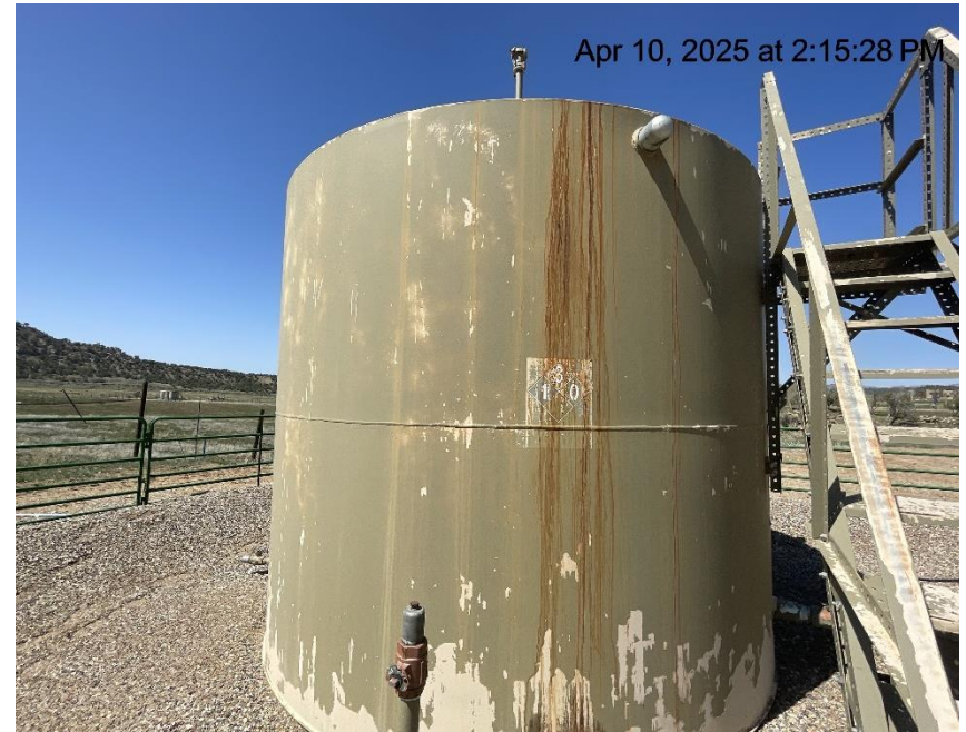
Photo # 481 Staining down side of tank
