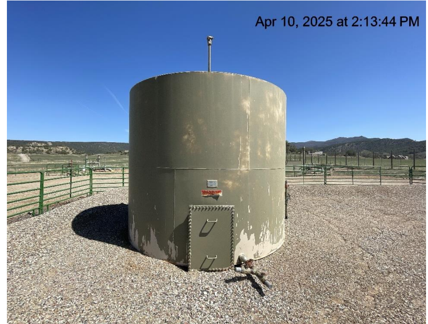
Photo # 477 Tank is disconnected & not in use/unused equipment
