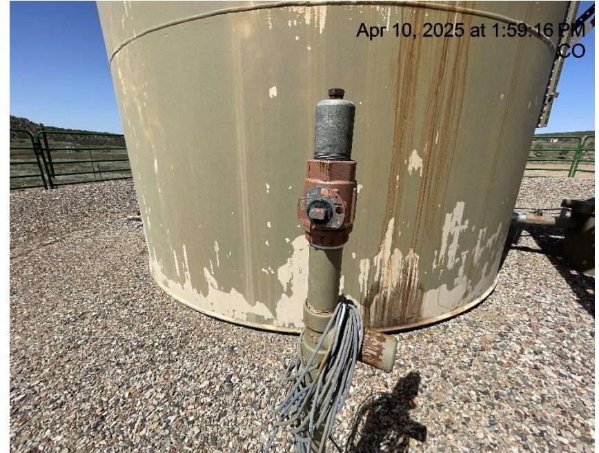
Photo # 475 Unused flowline lacks lockout tagout (OOSLAT)
