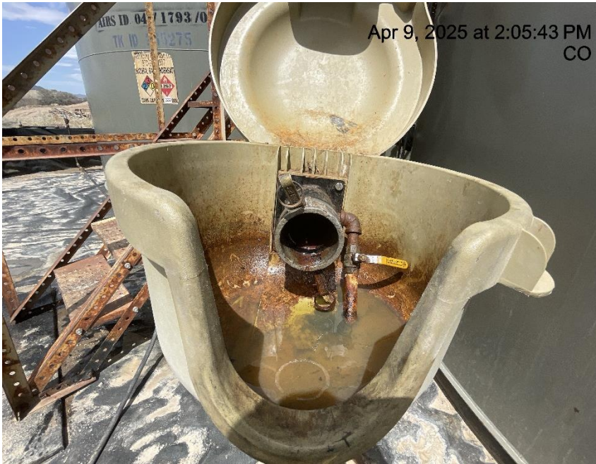
Photo # 9790 Open ended load line
