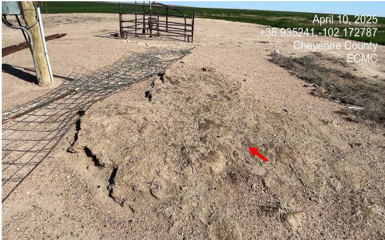
Photo 5. The pumpjack has been removed and there is hardened oil stained soil shown at red arrow. Also the fence panels need to be removed.
