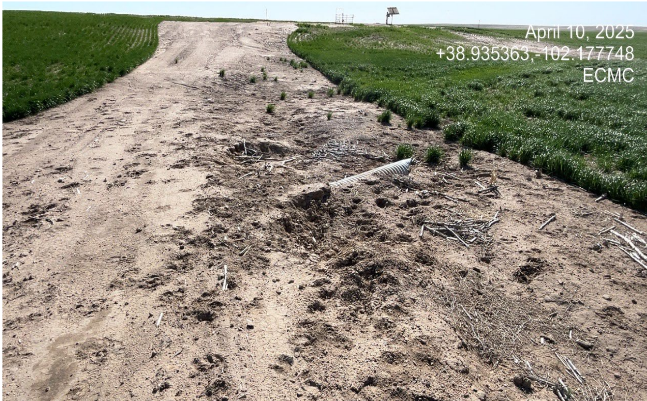
Photo 3. The culvert along the access road near the wellsite has washed out and needs to be repaired.
