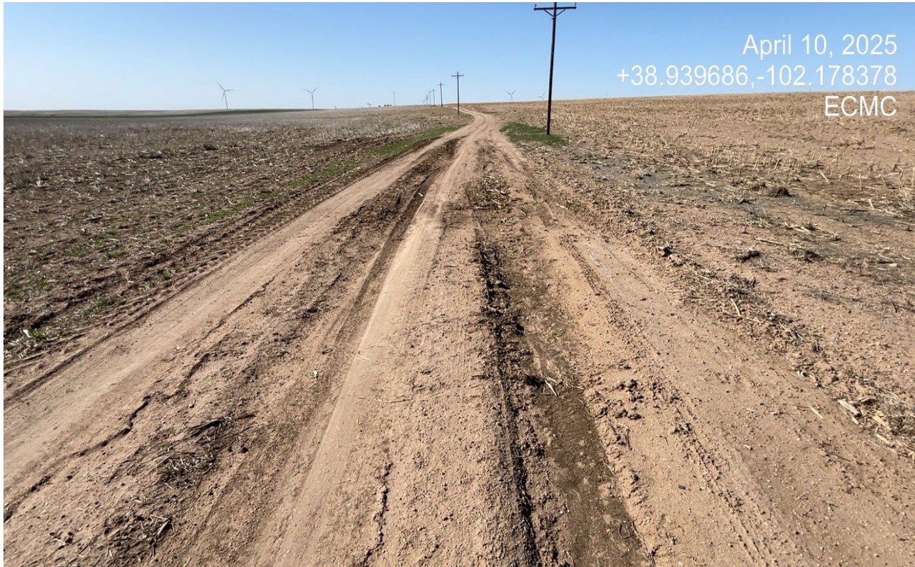
Photo 2. Facing south along the access road. The access road is rutted and not maintained in this area. Vehicle are widening the road at this area.
