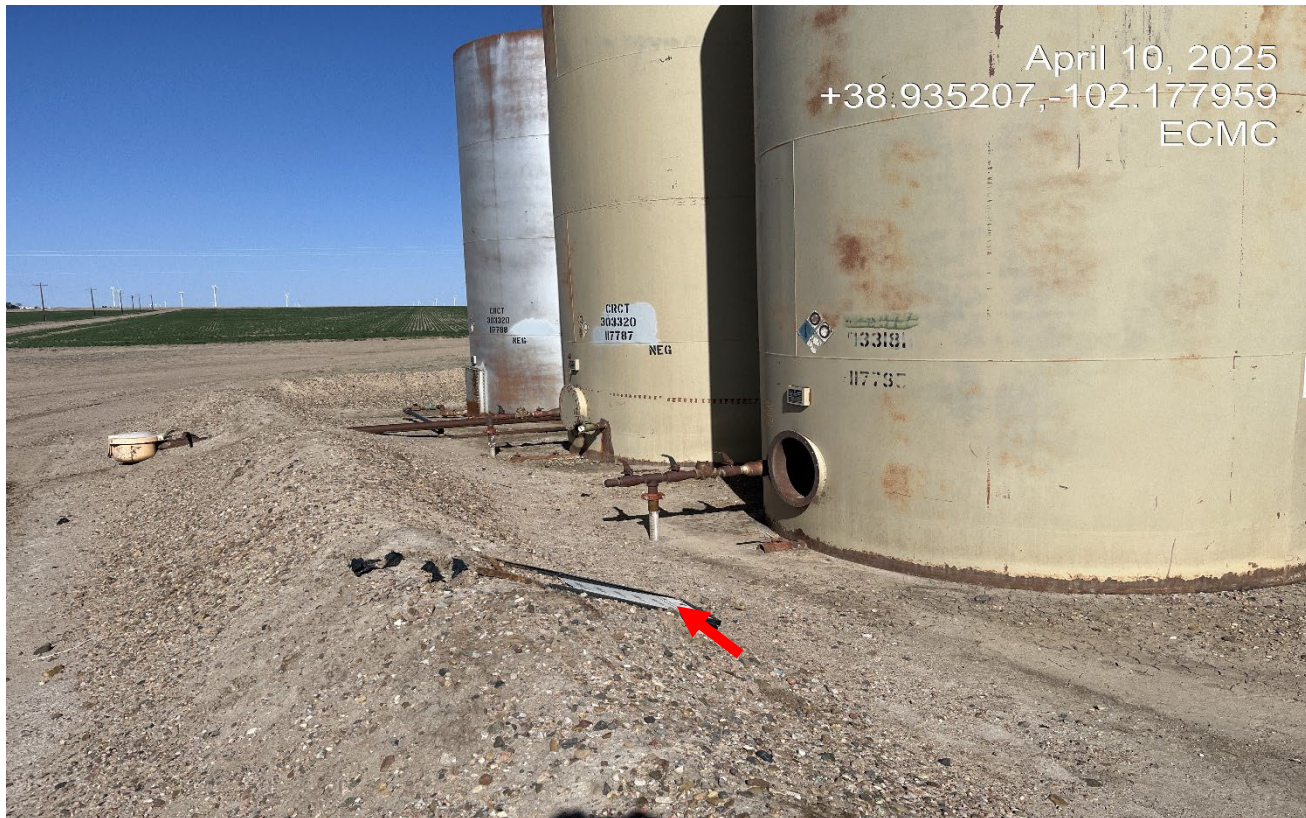
Photo 6. The tank battery sign has fallen over and the tank labels are faded.
