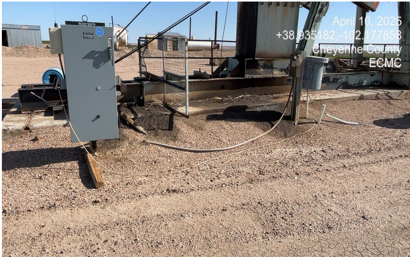
Photo 3. There are oil stained soils at the base of the pumpjack that need to be cleaned up and properly disposed.
