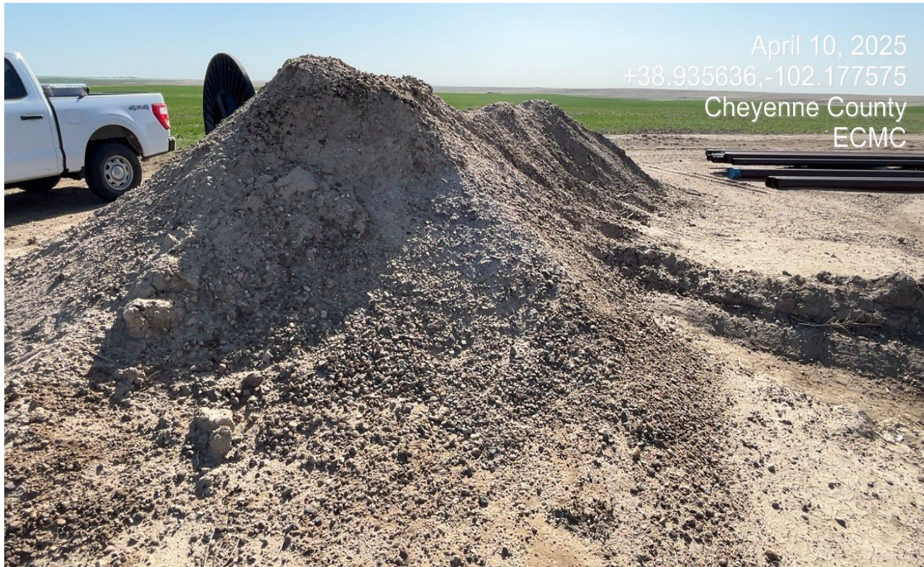
Photo 13. There is a pile of gravelly sand material stored at the northeast corner of the location. There is stained material incorporated into the pile. E&P waste must be stored with containment and liner.
