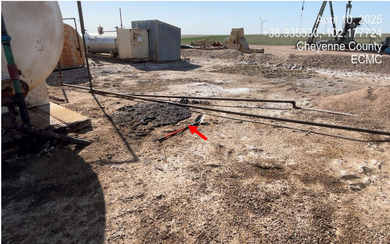
Photo 10. Facing southeast inside the tank battery. The is stained soil from a leak that occurred. The red arrow points to 4.5 ft. shovel for scale.
