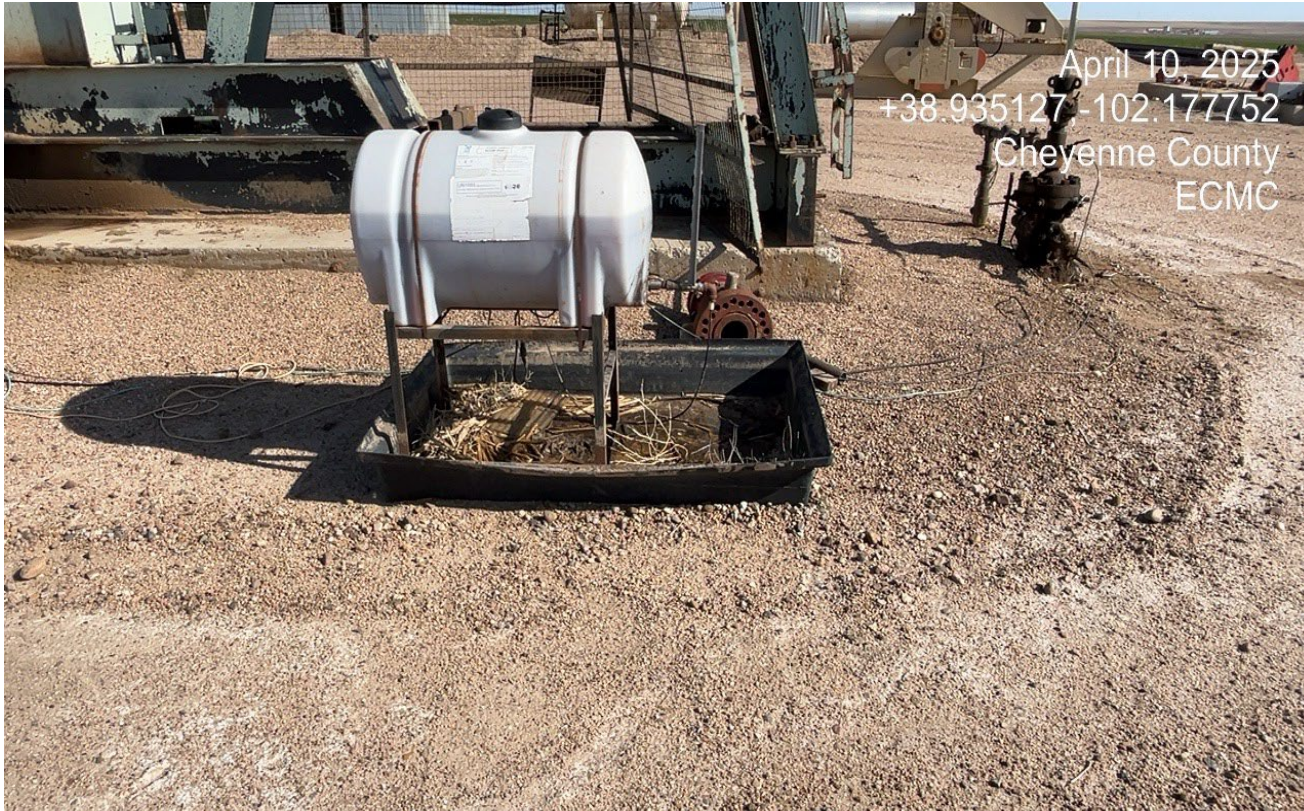
Photo 4. There is oily fluid in this secondary containment of the chemical barrel with no wildlife protections. This needs to be netted to prevent wildlife entry.
