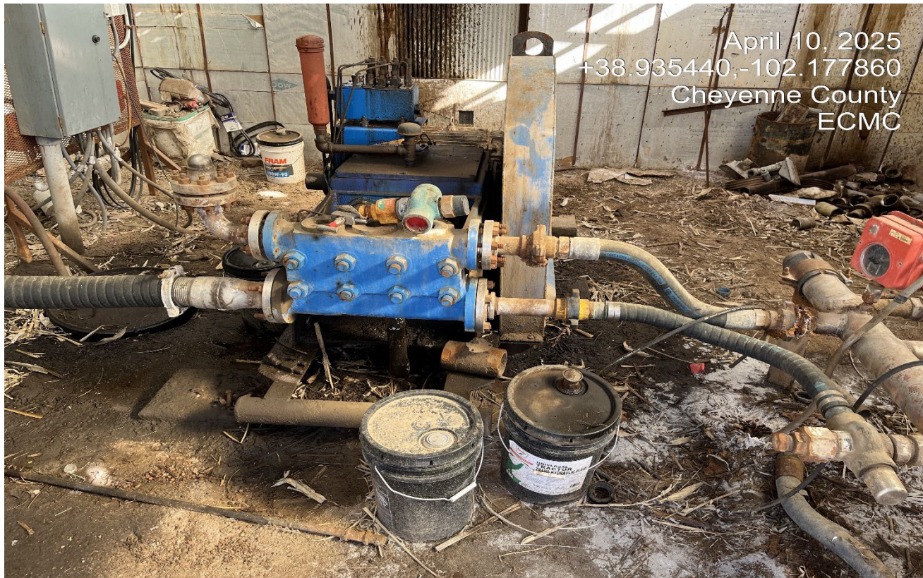
Photo 8. View of inside the shed shows oil stained soils and improper spill containment.
