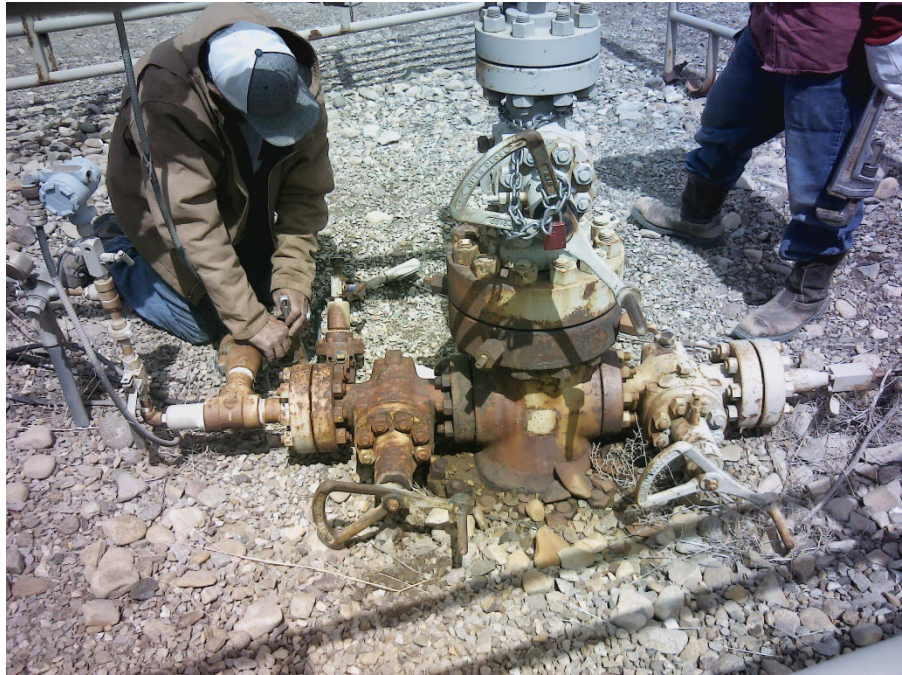
Wellhead during Bradenhead test. Wellhead leaking at tbg/csg head. See Optical Gas Imaging section.
