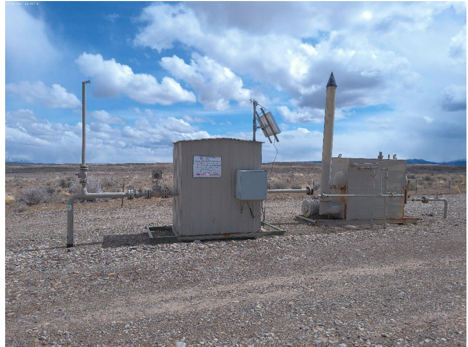
Separator and Meter housing
