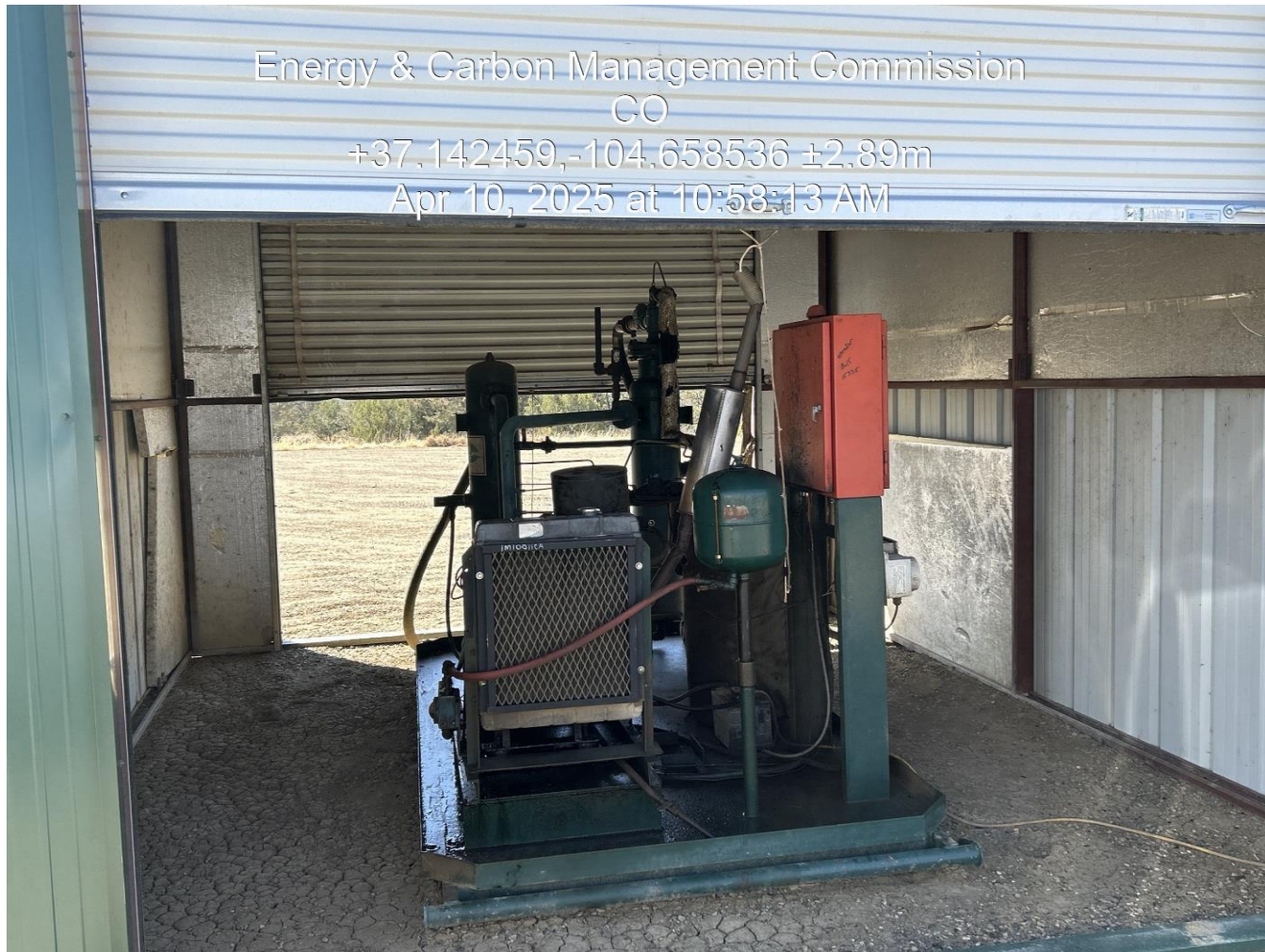
PHOTO 3: Compressor/Liquid Ring
