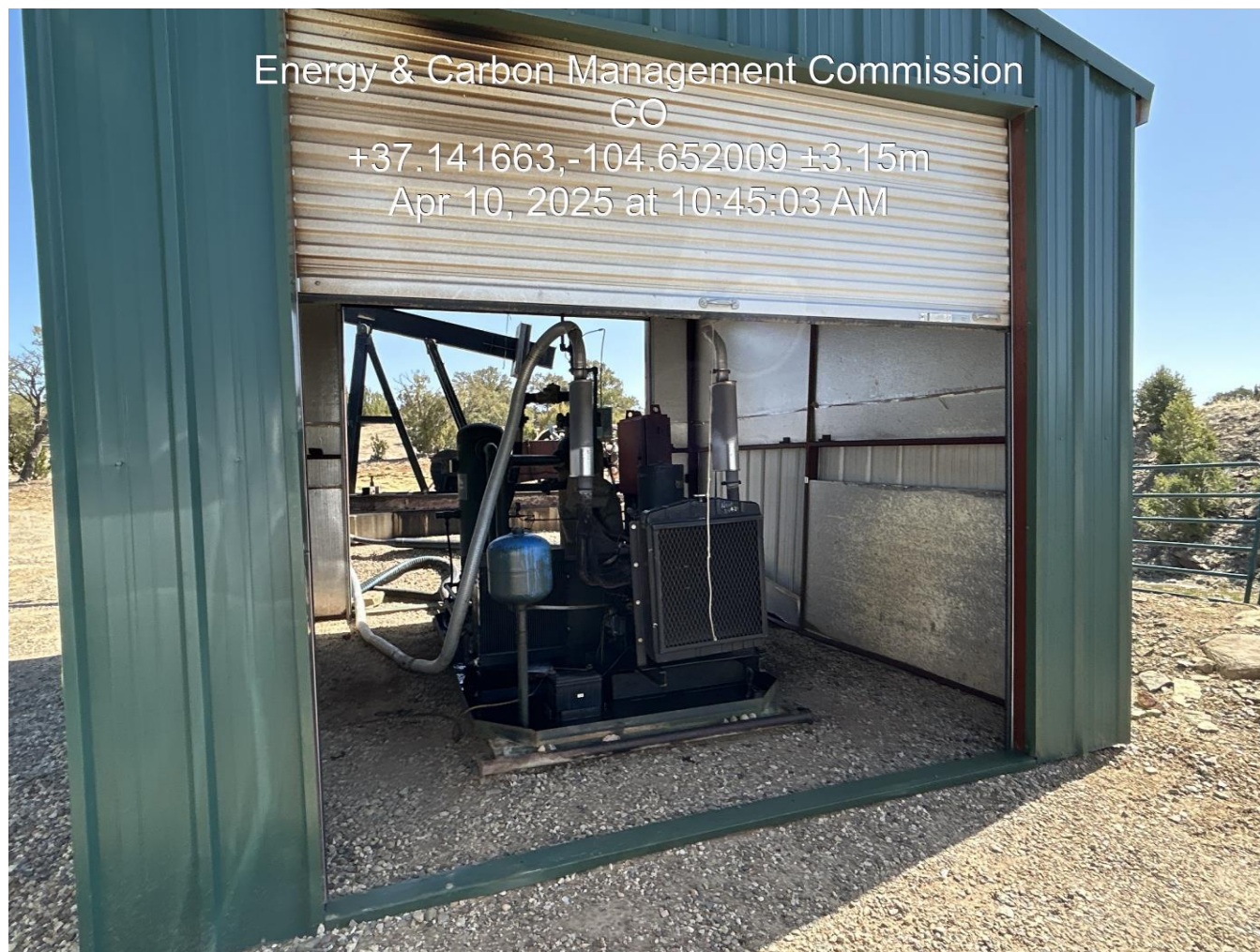
PHOTO 3: Compressor/Liquid Ring
