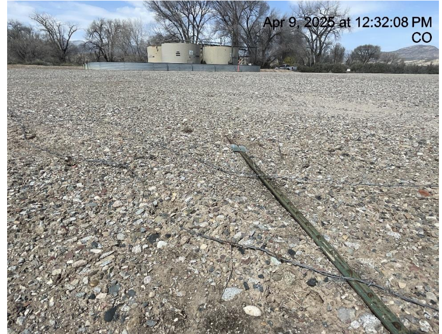
Photo # 9529 Barbed wire fence needs maintenance/wildlife hazard & trip hazard
