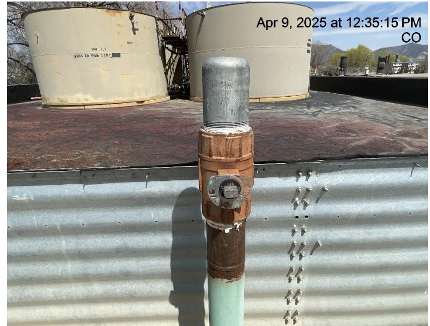
Photo # 9523 Unused flowline at tank battery lacks lockout tagout (OOSLAT)
