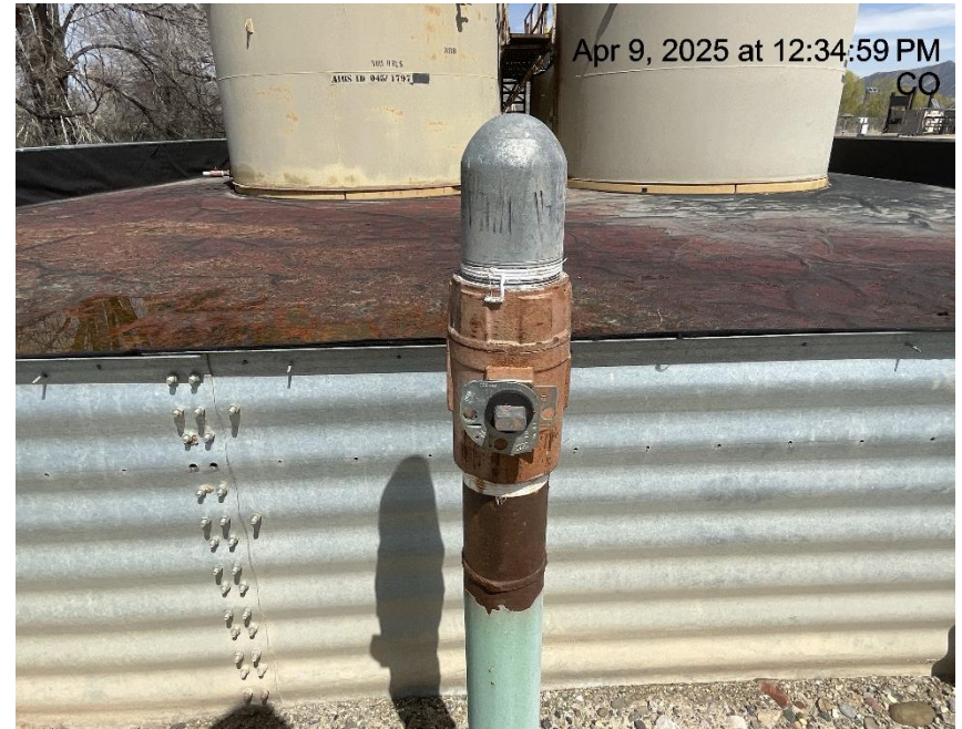
Photo # 9525 Unused flowline at tank battery lacks lockout tagout (OOSLAT)
