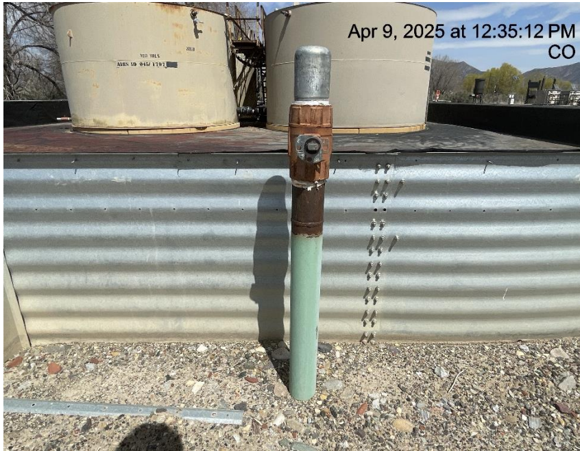
Photo # 9522 Unused flowline at tank battery lacks lockout tagout (OOSLAT)
