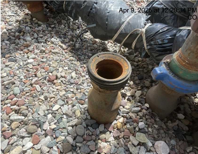
Photo # 9526 Unused flowline at separators lacks lockout tagout (OOSLAT) & additionally open ended line is a wildlife hazard/available for entry by wildlife
