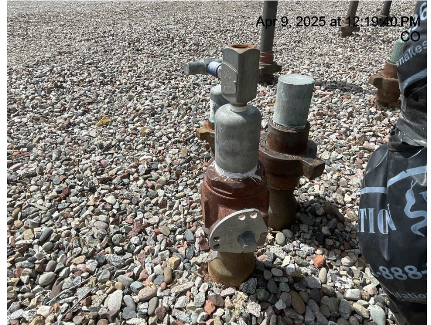
Photo # 9519 Unused flowlines at separators lack lockout tagout (OOSLAT)
