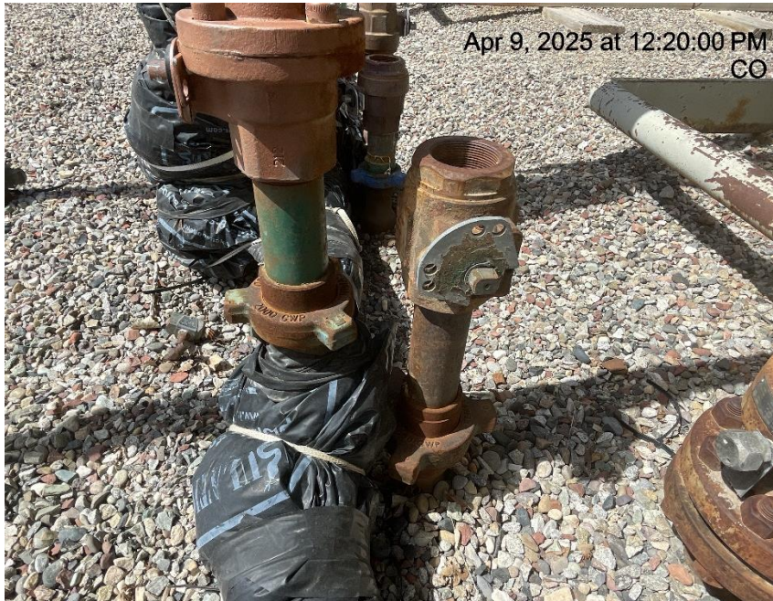
Photo # 9520 Unused flowline at separators lacks lockout tagout (OOSLAT)
