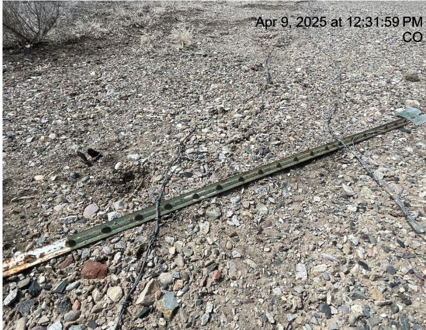
Photo # 9528 Barbed wire fence needs maintenance/wildlife hazard & trip hazard
