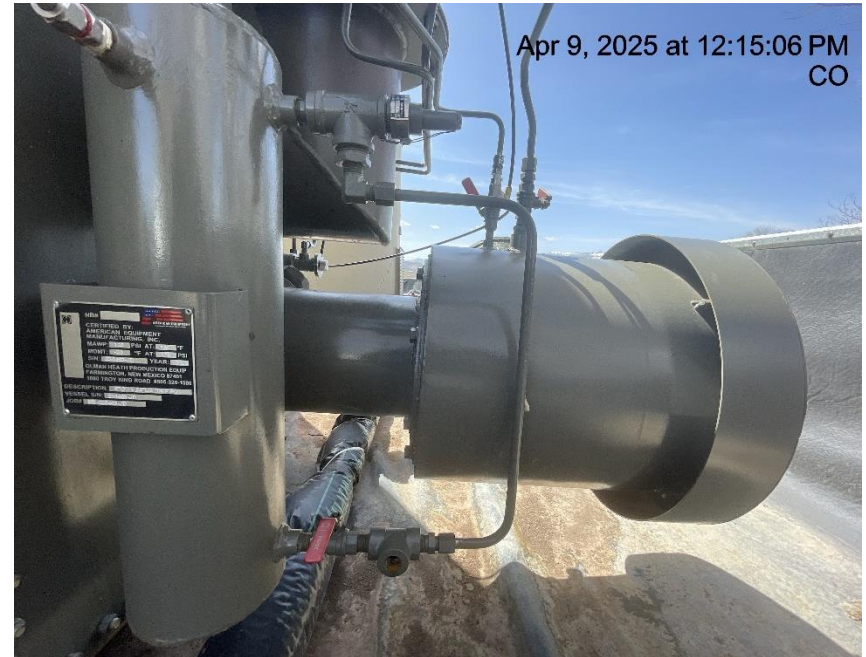
Photo # 9533 PRV vent line does not comply with CECMC pressure safety device rules or general safety rules
