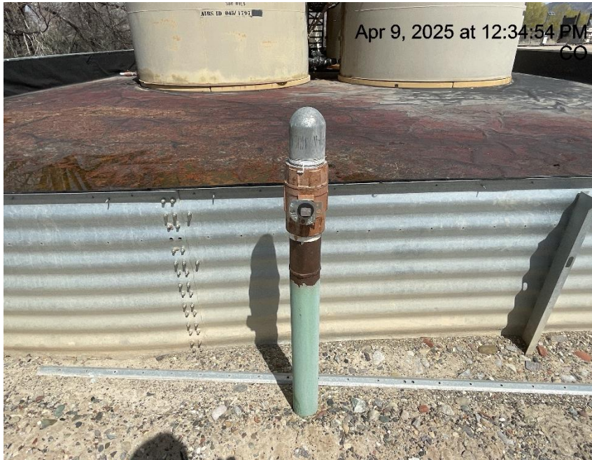
Photo # 9524 Unused flowline at tank battery lacks lockout tagout (OOSLAT)
