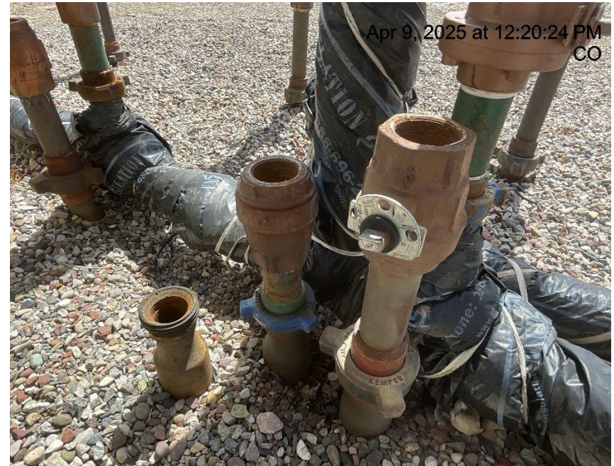
Photo # 9521 Unused flowlines at separators lack lockout tagout (OOSLAT) & additionally open ended line is a wildlife hazard
