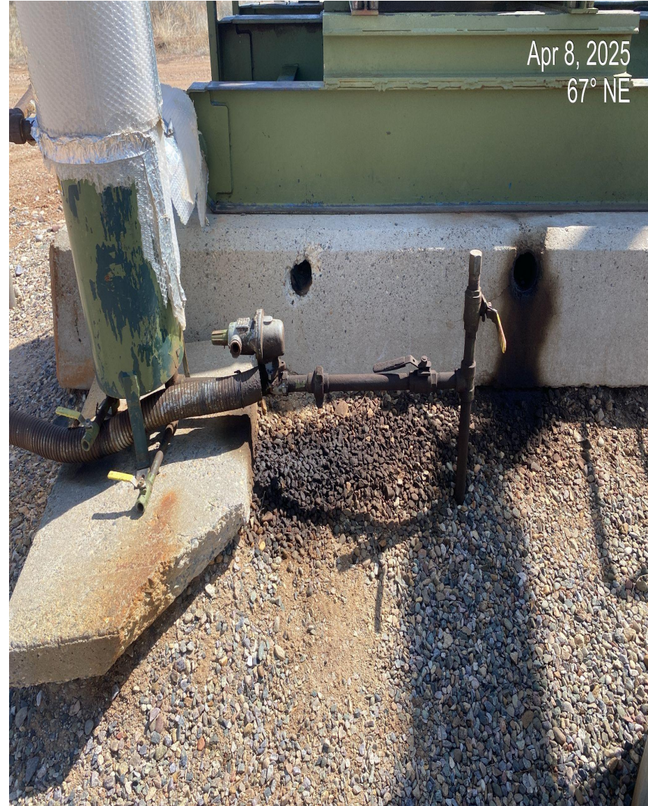
Photo 2. Stained soils at pump jacks and mufflers.
