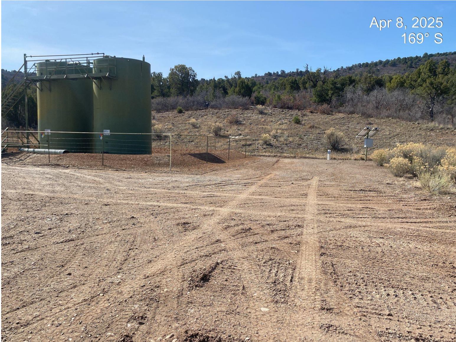
Photo 2. Rutting issues on active pad have been addressed/resolved.
