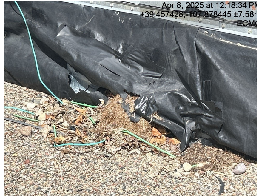
Holes in containment
