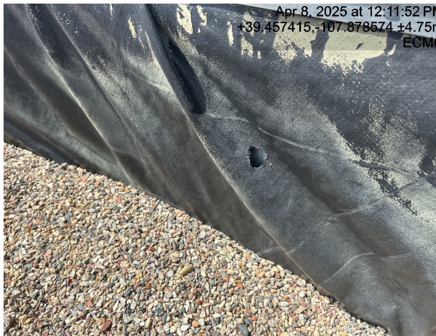
Holes in containment
