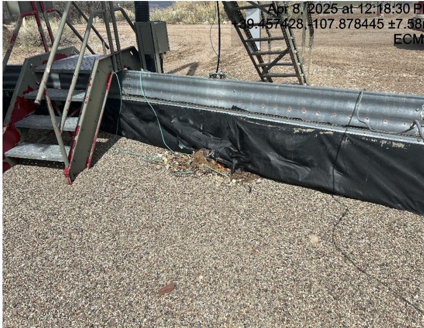
Holes in containment
