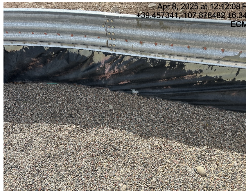
Holes in containment
