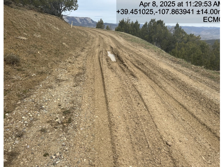
Lack of stabilization/compaction on access road
