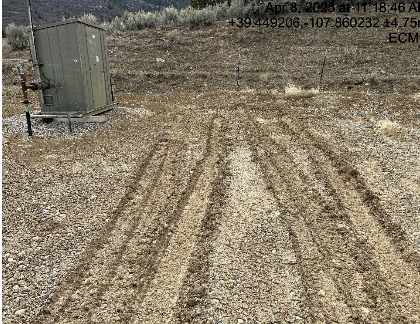
Lack of stabilization/compaction/tracking controls
