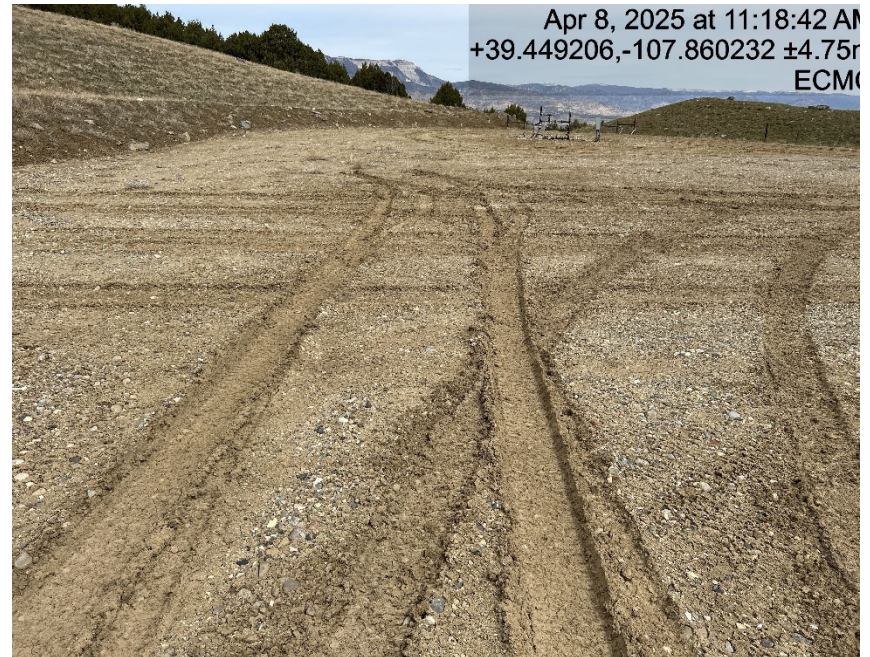
Lack of stabilization/compaction/tracking controls
