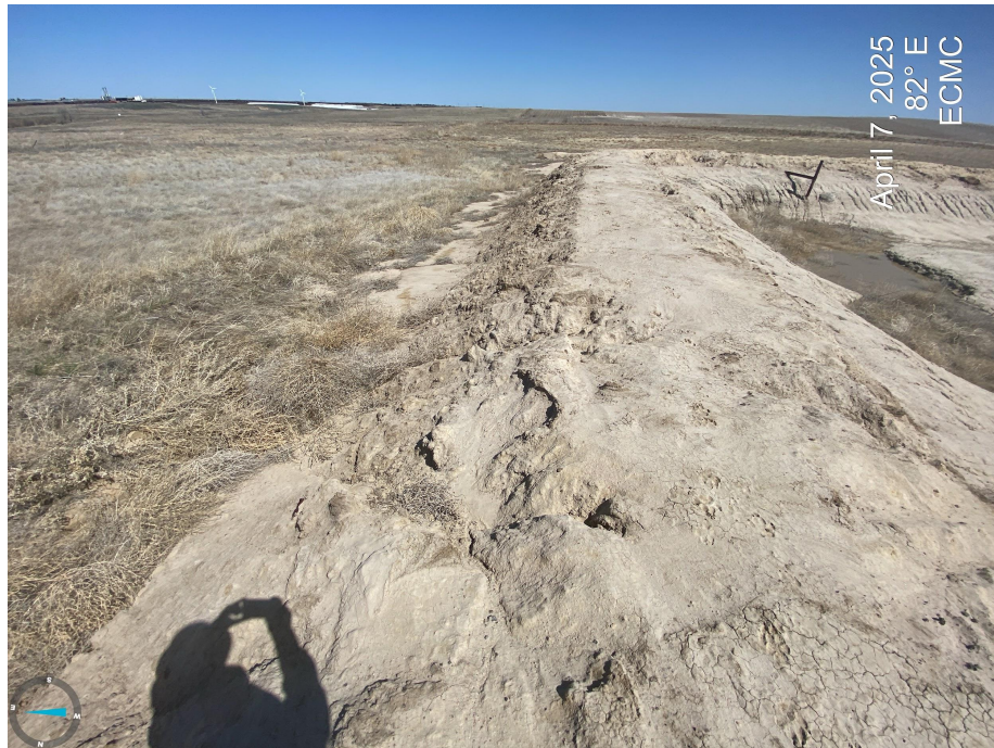
Photos 13 & 14. Unstabilized soils and erosion degradation evident at pits. Undesirable vegetation observed throughout pits.
