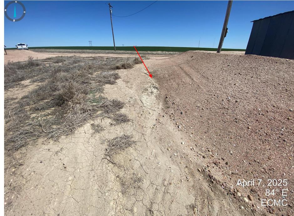
**Photos 5 & 6.** Photo 5 (left) illustrates that a perimeter ditch has been installed along the western portion of the location. Photo 6 (right) illustrates that erosion degradation previously observed near the separator does not appear to have been repaired or stabilized.
