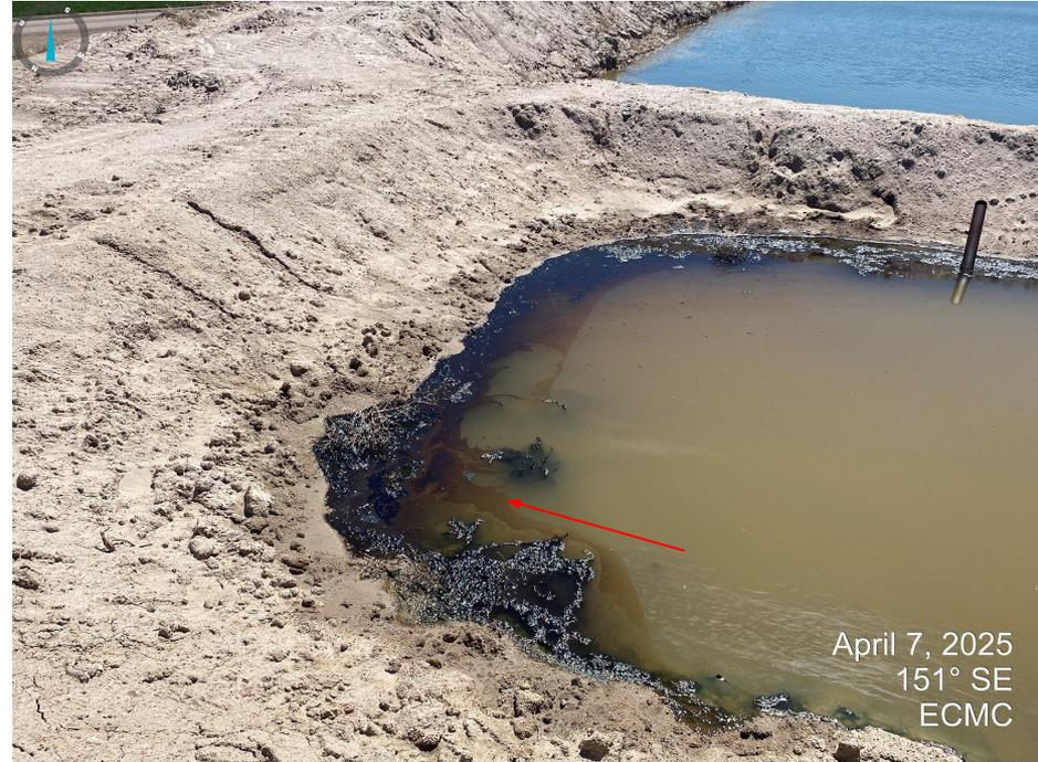
**Photos 11 & 12.** Visible hydrocarbons observed on the surface of skim pit with visible sheen evident.
