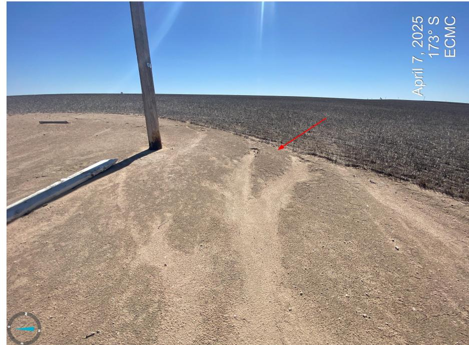
**Photos 13 & 14.** Erosion degradation previously observed near the well location does not appear to have been repaired or stabilized to prevent reoccurrence.
