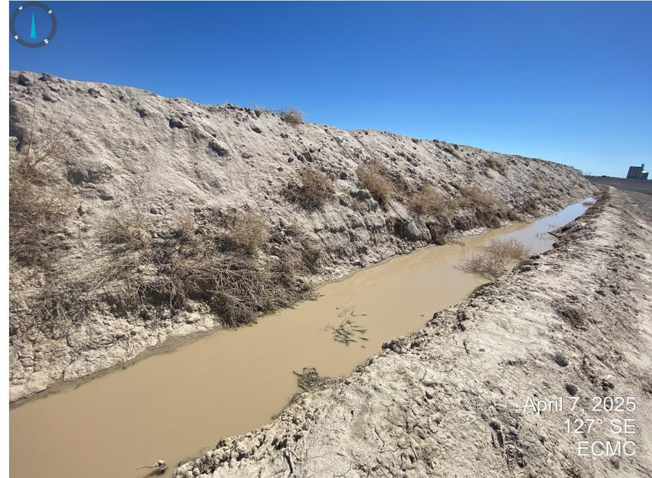
**Photos 7 & 8.** Photos illustrate that perimeter stormwater controls appear to be properly functioning. Photo 8 (right) illustrates weedy debris on pit walls.
