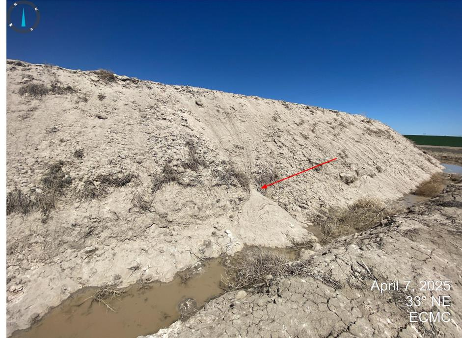
**Photos 9 & 10.** Evidence of erosion degradation observed at the pit walls.
