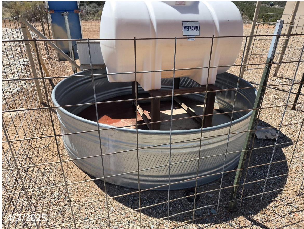
Photo 3: Wildlife protection BMPs missing or insufficient at secondary containment.
