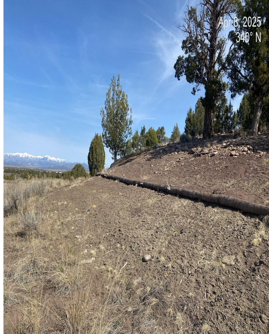
Photo 2. Location cut slope/eastern interim reclamation area remains with mostly bare soils. Additional reclamation/seeding efforts are needed in this area. Wattle BMPs are functioning at this time.
