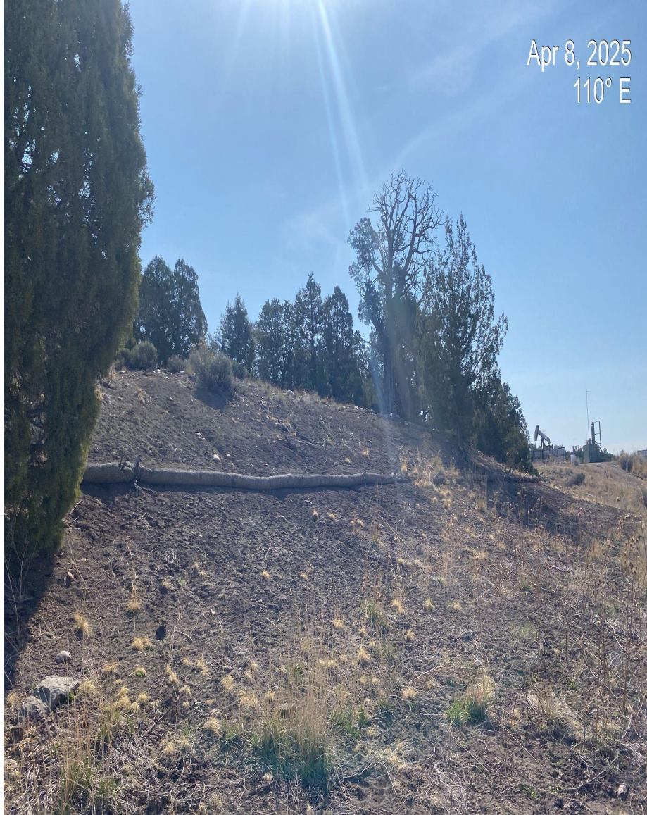
Photo 2. Location cut slope/eastern interim reclamation area remains with mostly bare soils. Additional reclamation/seeding efforts are needed in this area. Wattle BMPs are functioning at this time.
