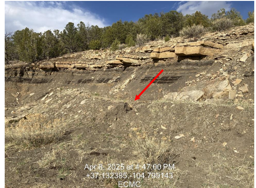
Photo 8 – Breach in BMP, stormwater overtopping BMP
