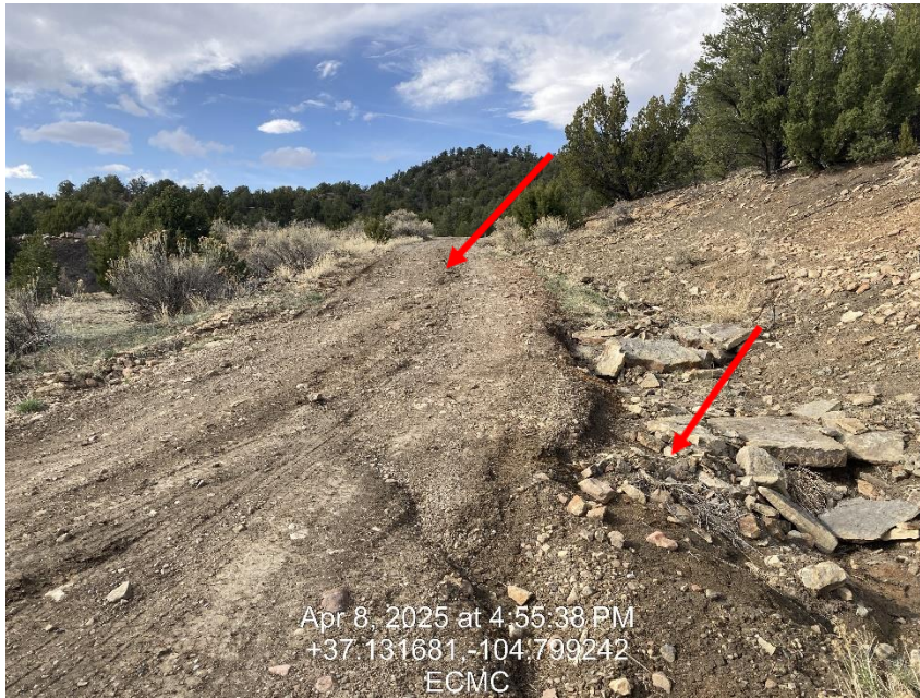
Photo 9 – Stormwater running down access road
