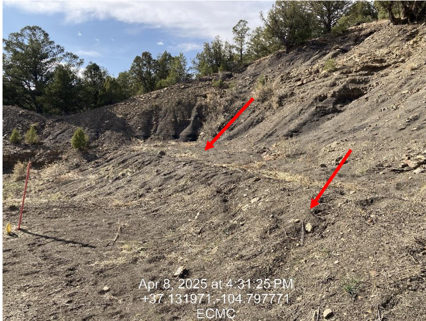
Photo 9 – BMP's full, Stormwater overtopping BMP's
