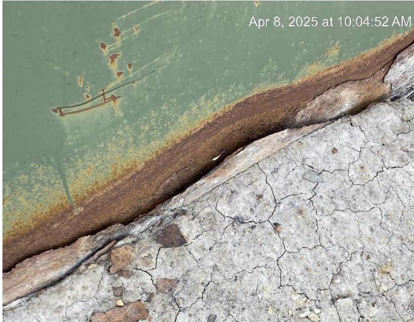
Hole in containment
