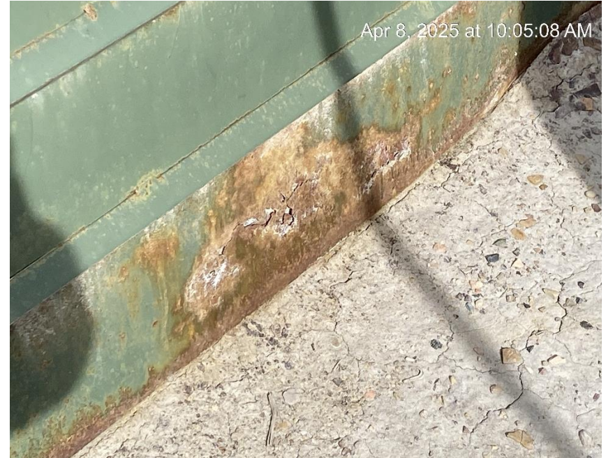
Containment damage
