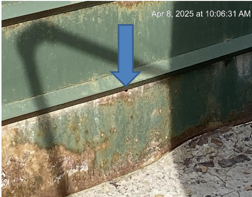
Hole in containment
