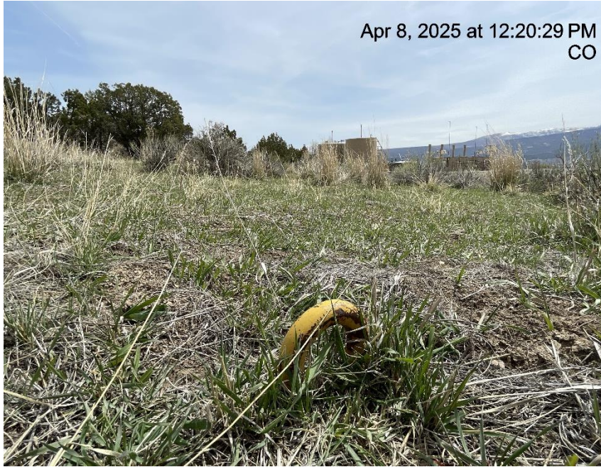
Photo # 9284 Unmarked deadman
