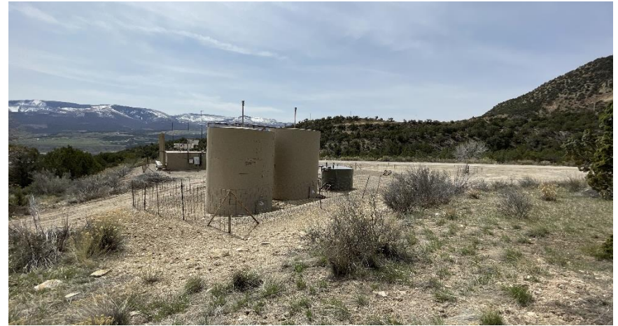
North East corner of location.
