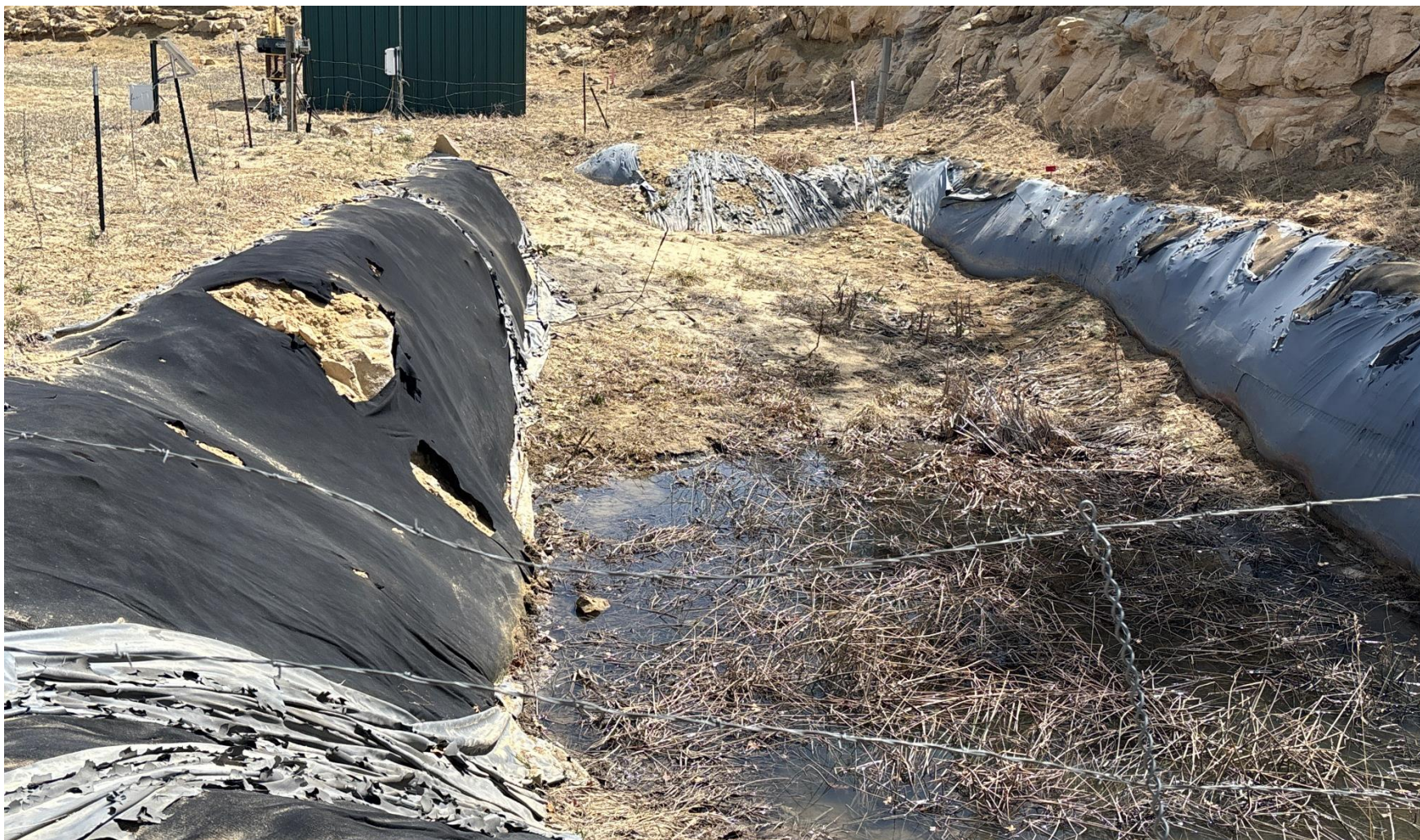
PHOTO 4: pit liner compromised (Rule 910). Reduce fluid level in pit, contact ECMC EPS staff for directives. CA DATE 4/9/2025.
