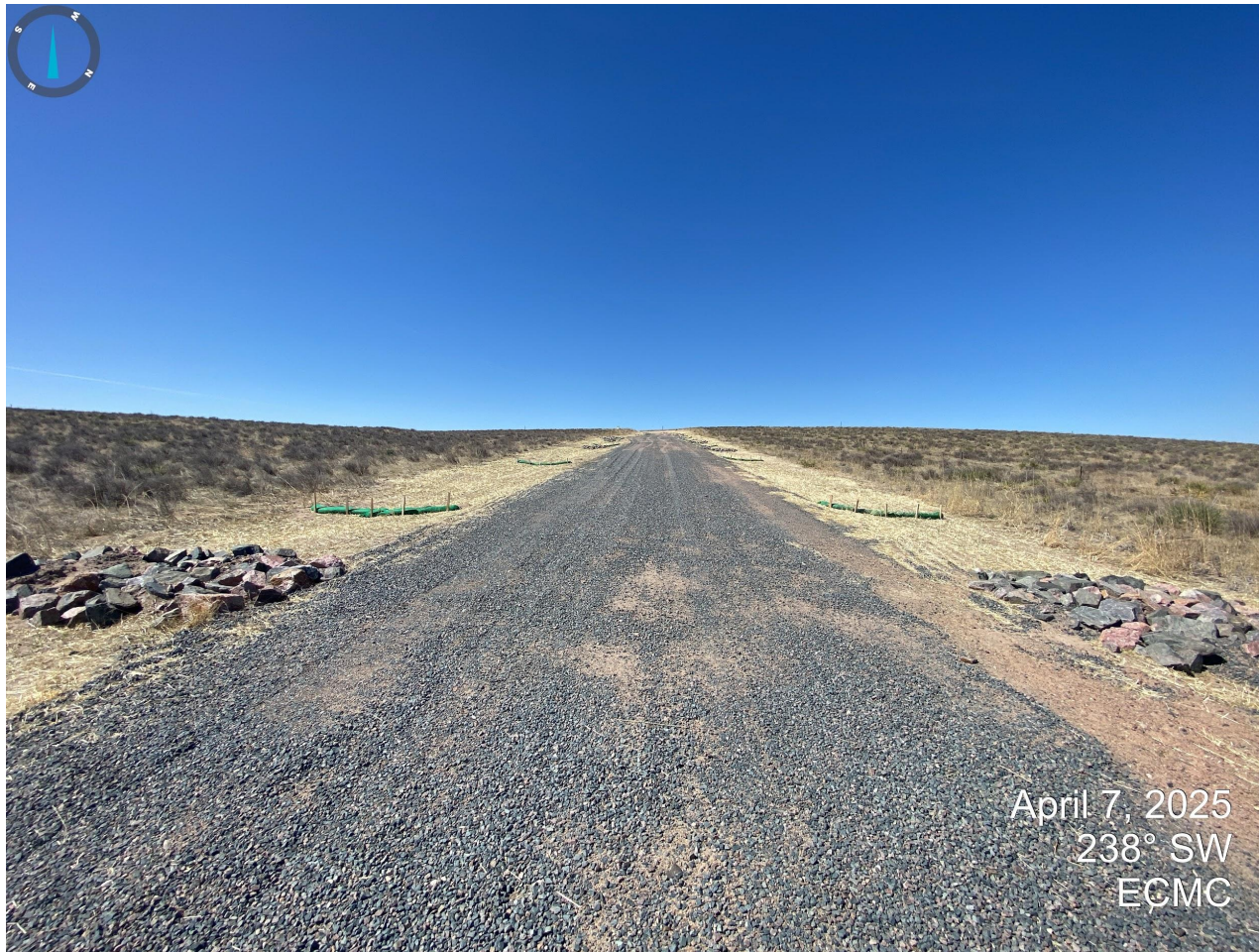
Photo 13. Taken along the access road. It appears that stormwater control measures have been maintained, erosion degradation has been repaired, and unstabilized soils were drill seeded and mulched.
