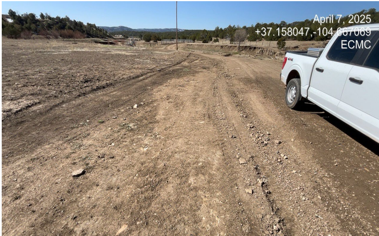
Photo 2. Facing back toward the repair along the road side. This area of the road may need additional BMP's such as rock check dams.
