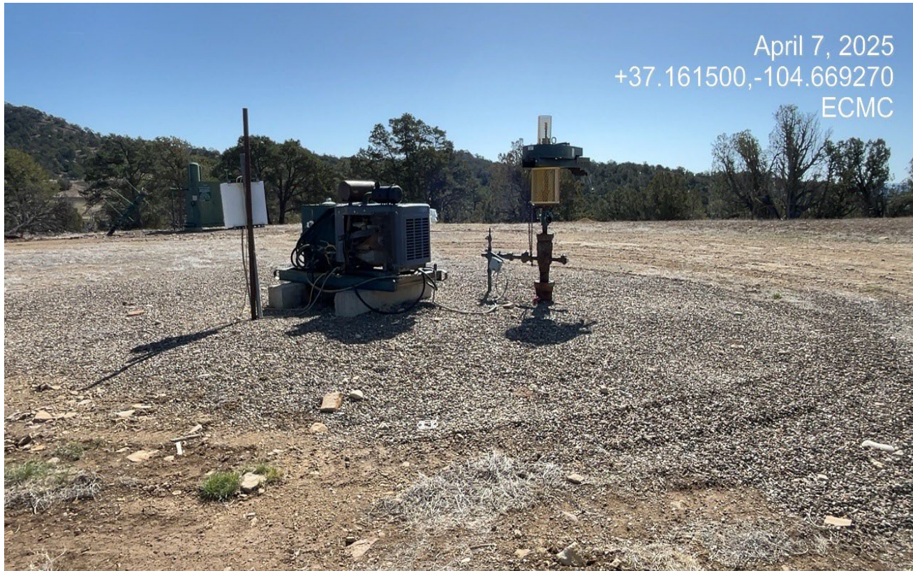
Photo 4. Facing southeast at the wellsite.
