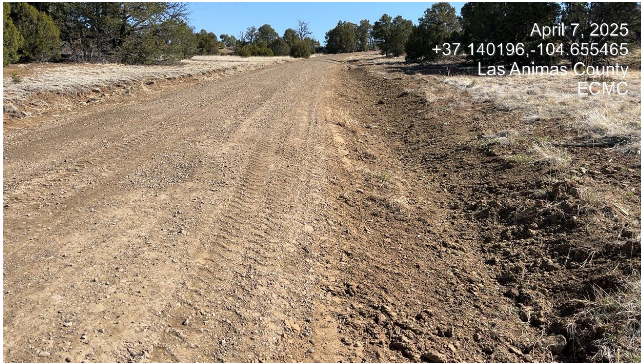
Photo 3. Facing northeast along the access road . This area has been repaired and reseeded. This area may need additional BMP's.
