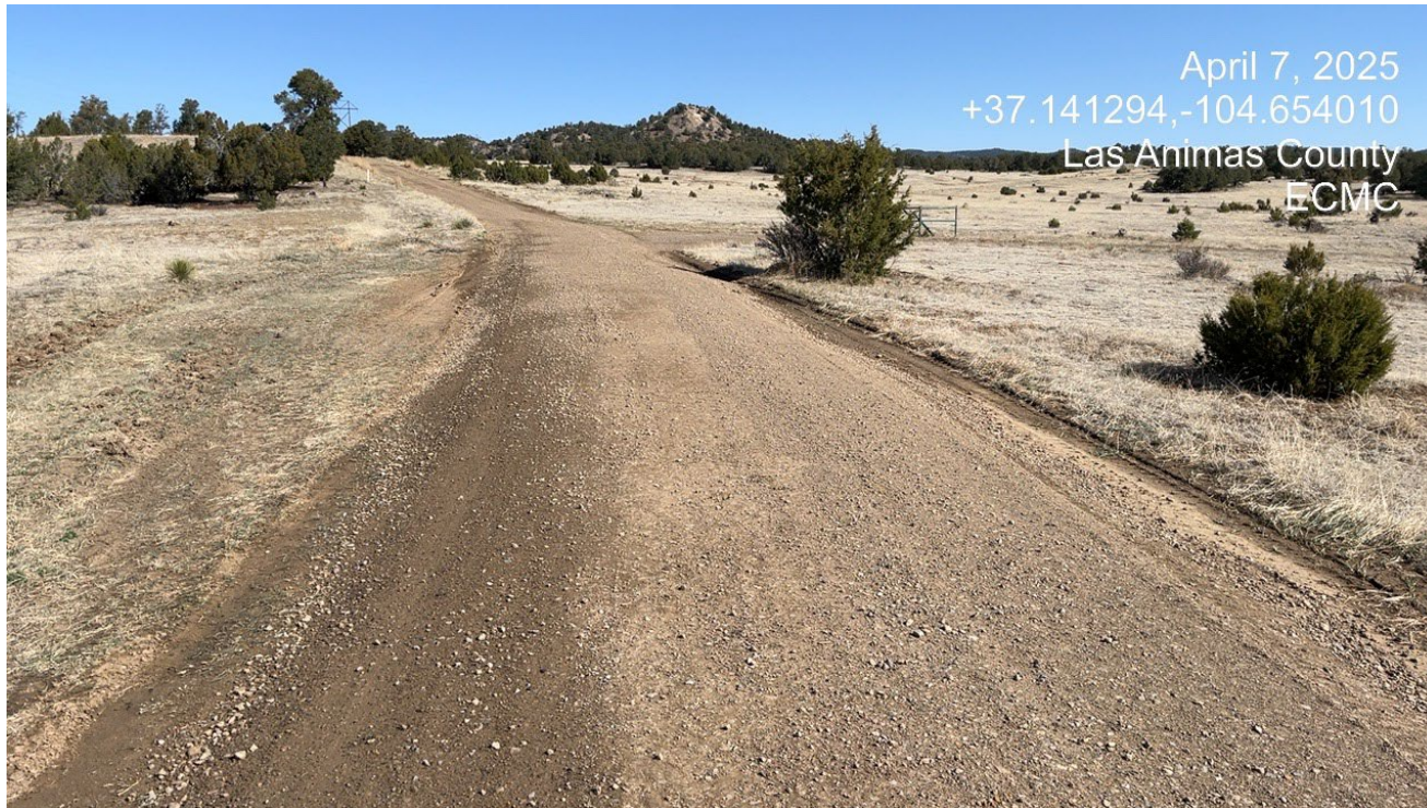
Photo 4. Facing north along the access road. This area has been built up with roadbase and crowing of the road.
