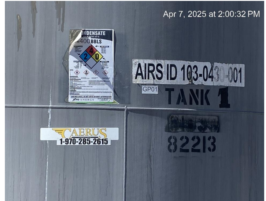
Replace when damaged
