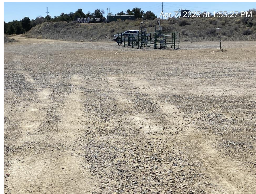
Well pad from South entrance
